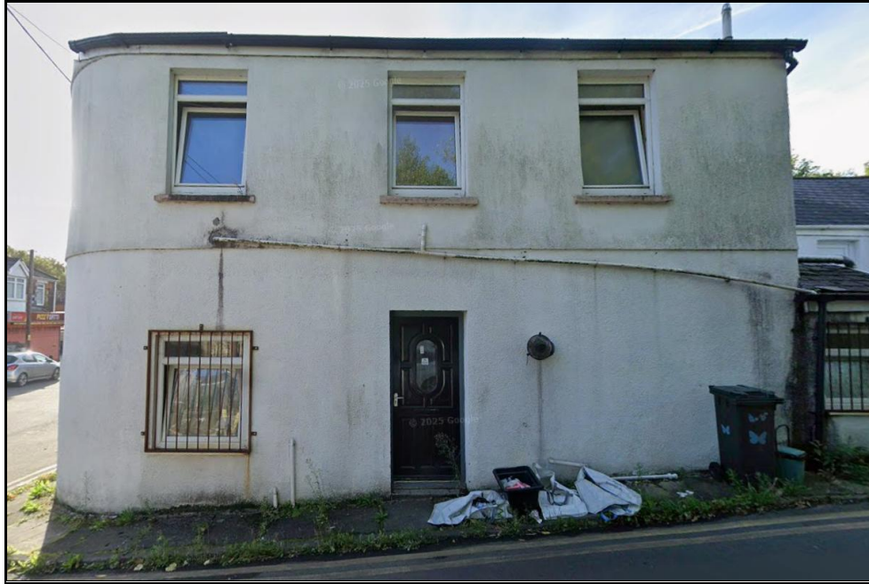
Photograph 2 – Rear Elevation of 9 High Street
