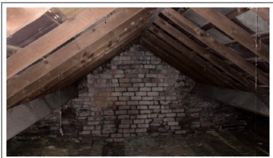
Photo 5: Typical view in the unlined roof void
