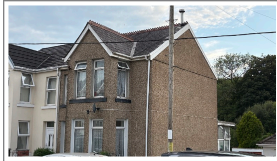
Photo 2: East/North facing elevations
