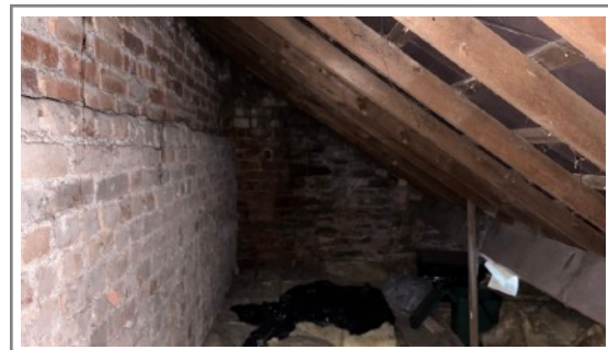
Photo 6: General view of the roof void area looking north
