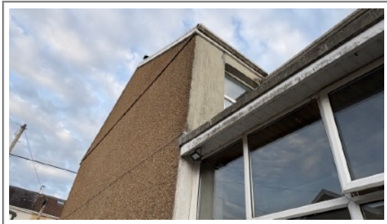
Photo 3: North facing elevations (detail)
