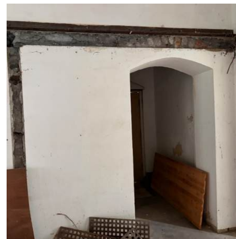
Figure 11 - Doorway to porchway
