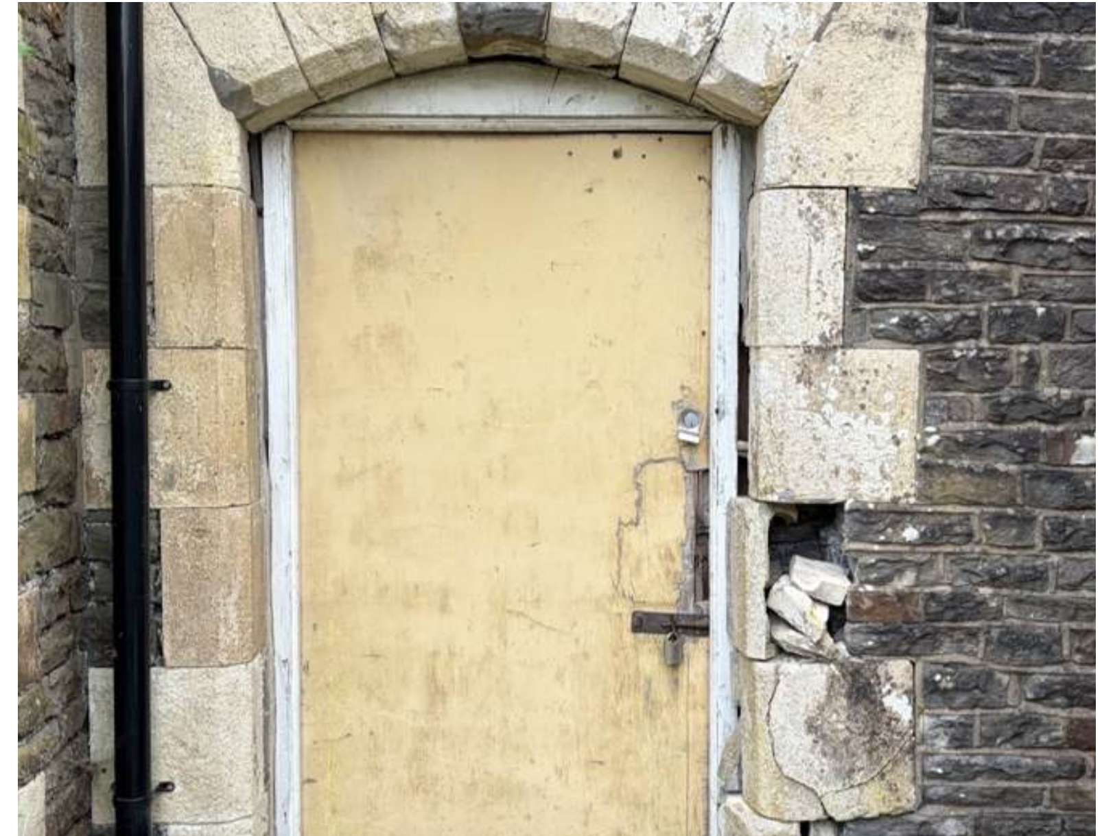
Figure 14 – Failed stonework
