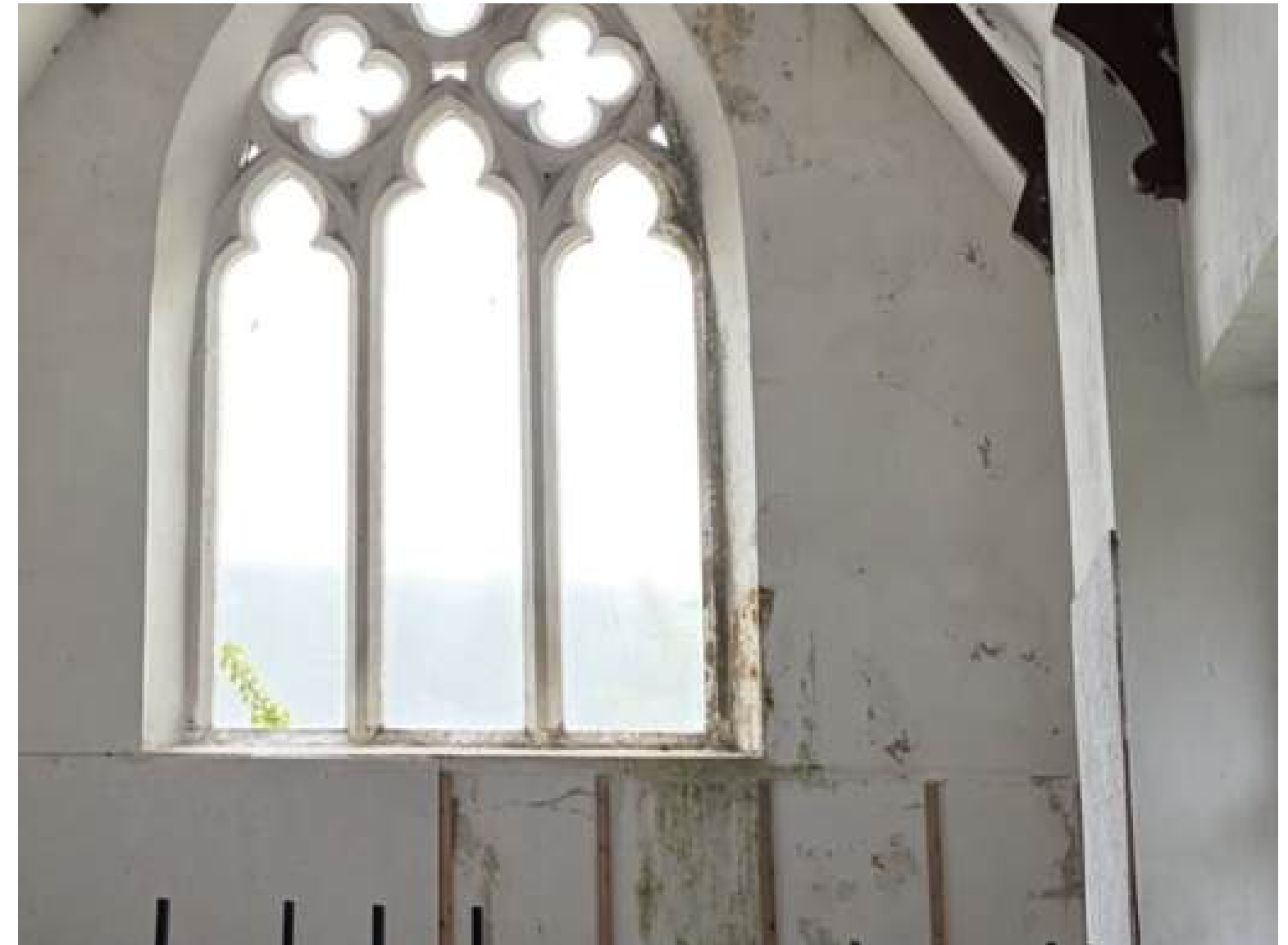
Figure 24 - Water ingress
