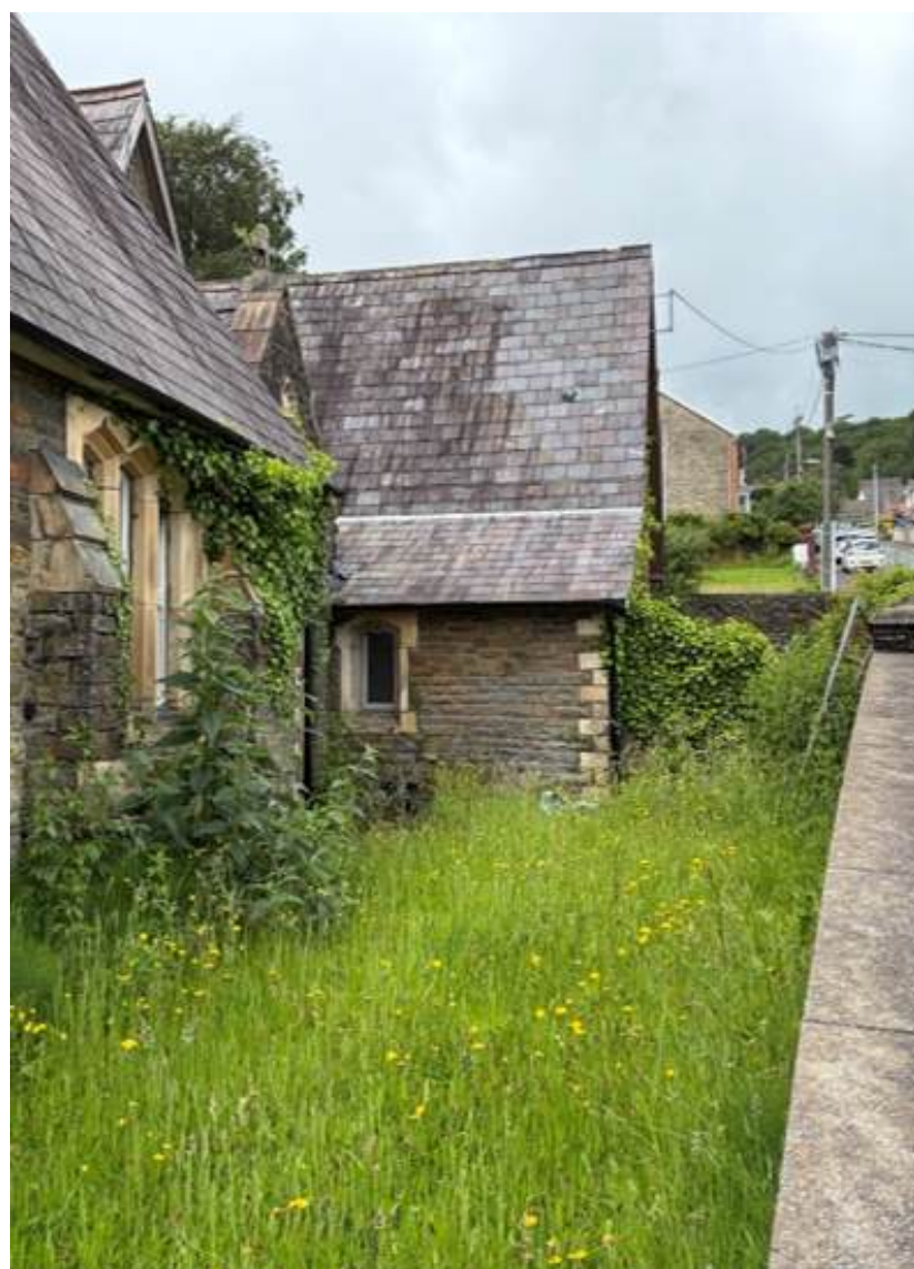
Figure 6 - South west elevation and gable
