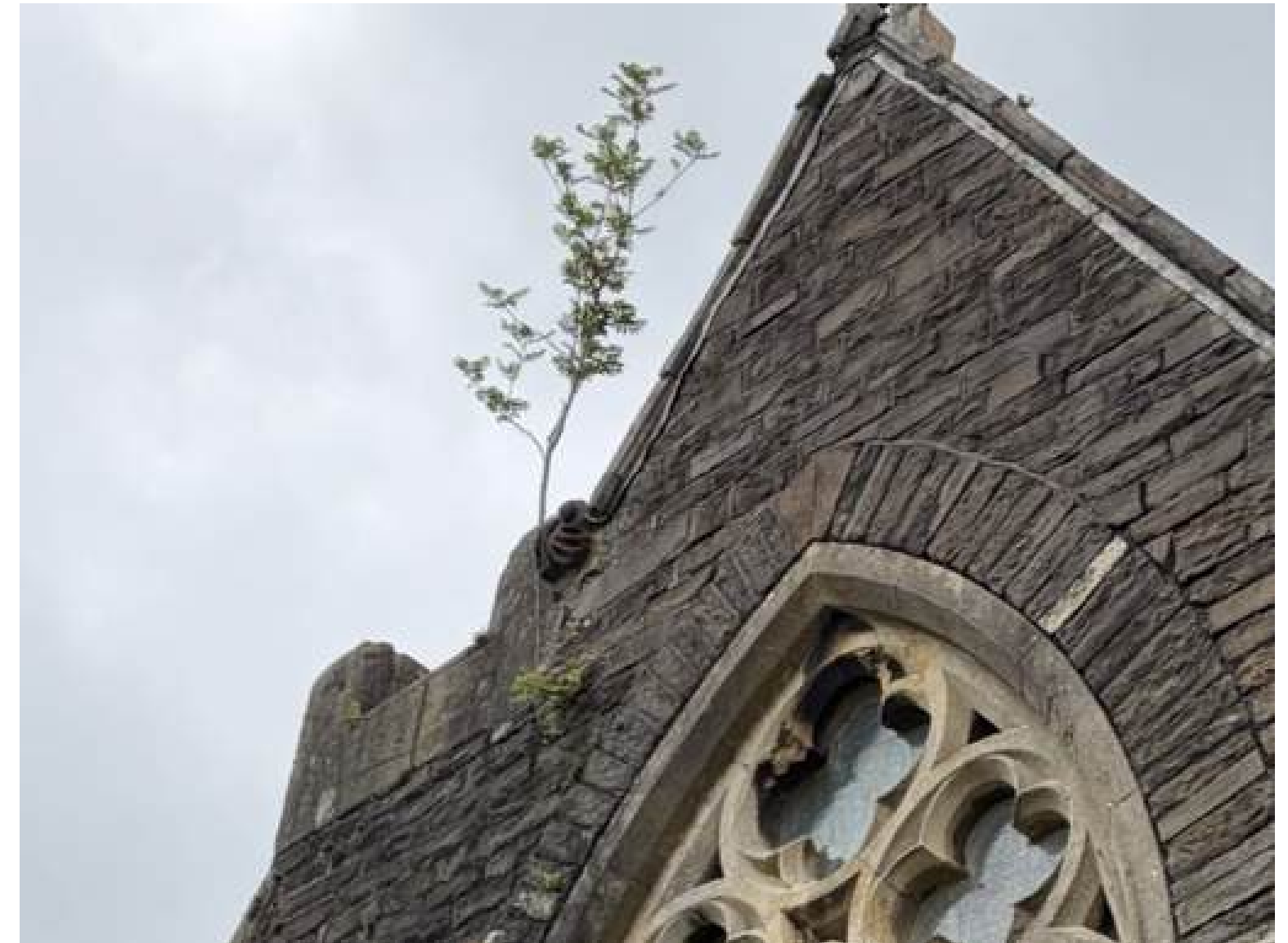
Figure 16 - Foliage growth and stone defects
