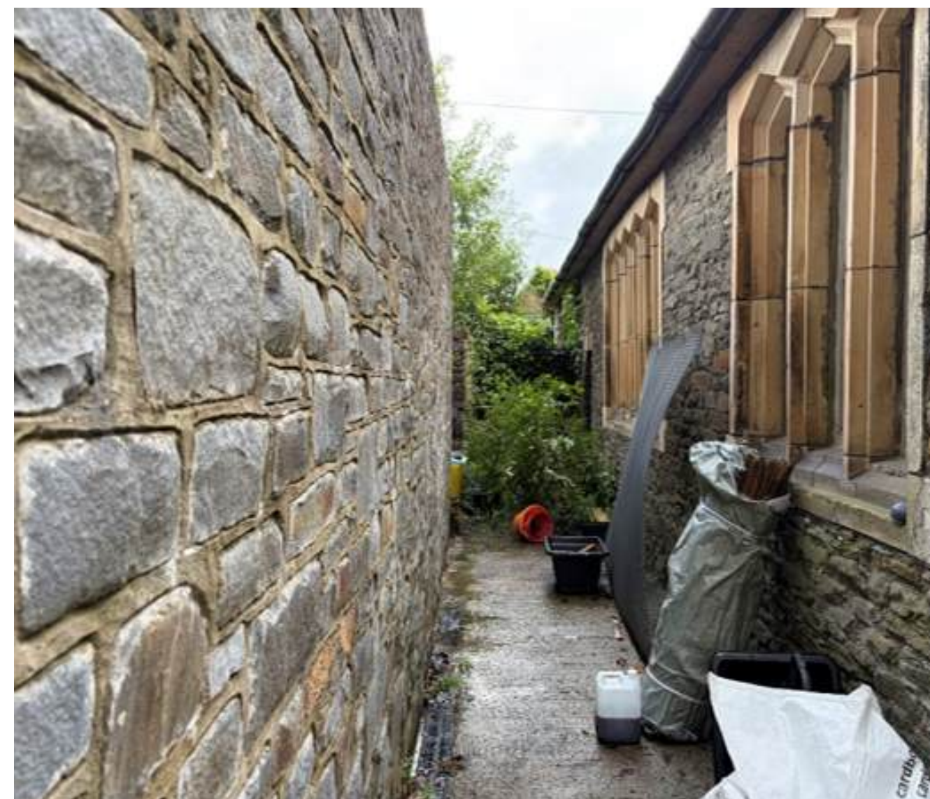
Figure 7 - South east elevation
