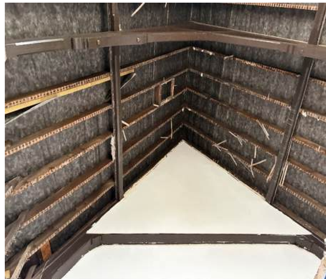
Figure 22 - Missing ceiling
