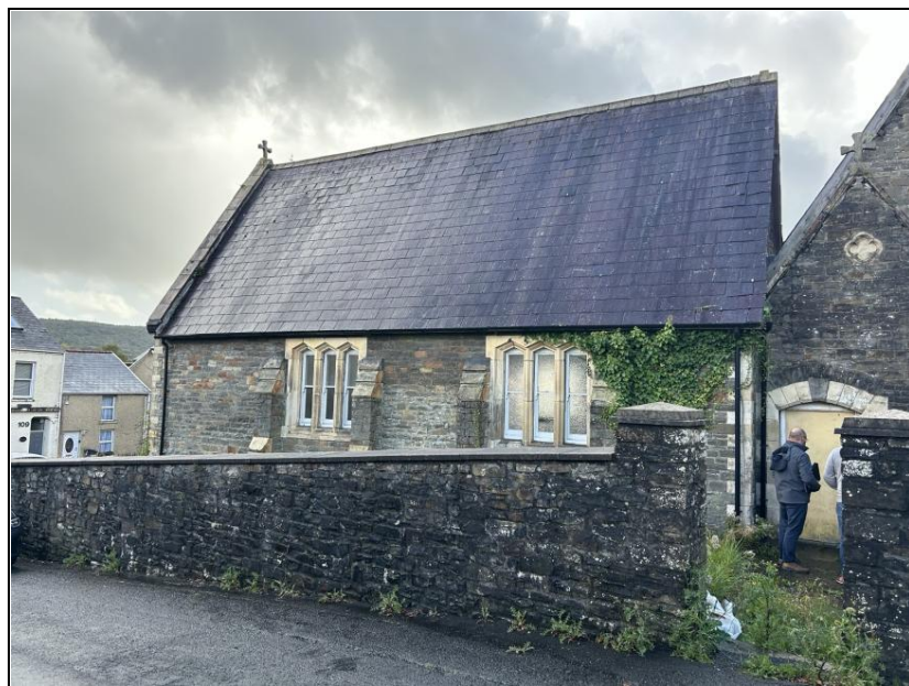
Photograph 6 – Eastern (Rear) Elevation and Proposed Access Point to Community Hub
