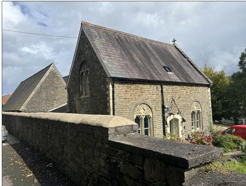
Photograph 3 – Front and Northern Elevations
