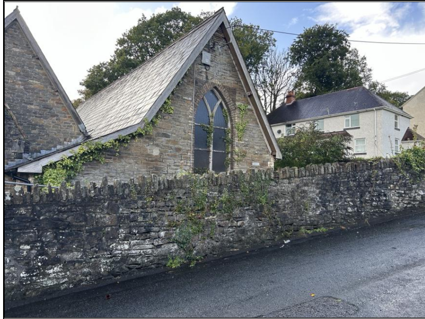
Photograph 5 – Eastern (Rear) Elevation
