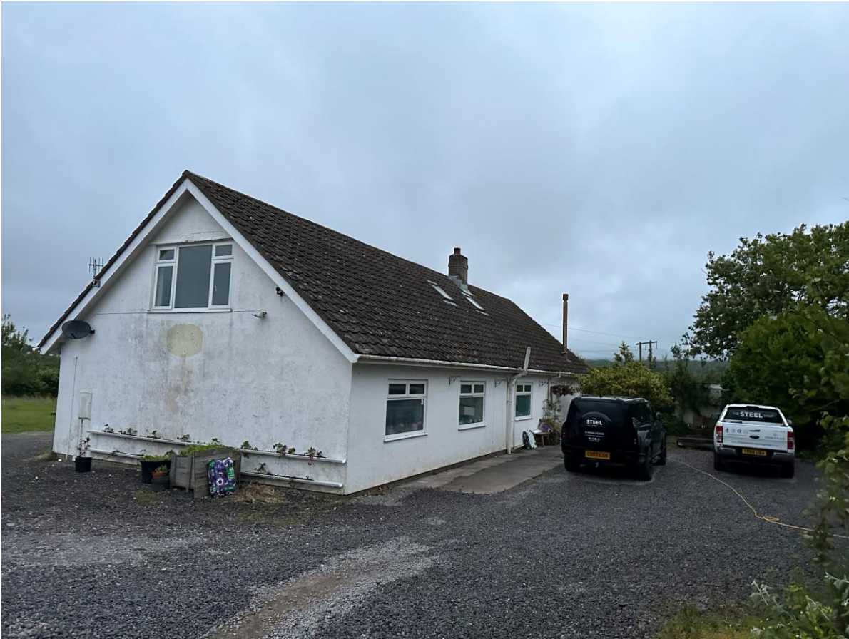
Plate 1. Existing dwelling and crushed-stone driveway / hardstanding, corresponding broadly with TN6 and TN8.
