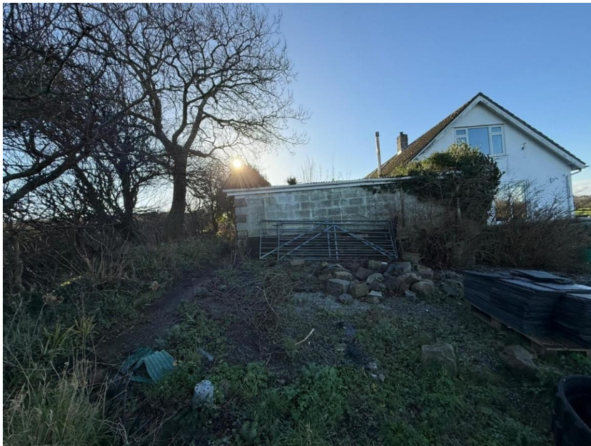
Figure 11: Side elevation and view of garage
