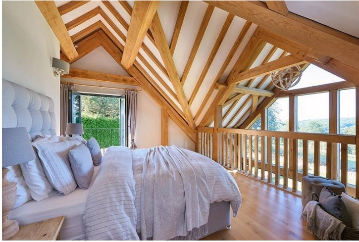
Figure 26: Internal vaulted spaces with exposed oak framework
