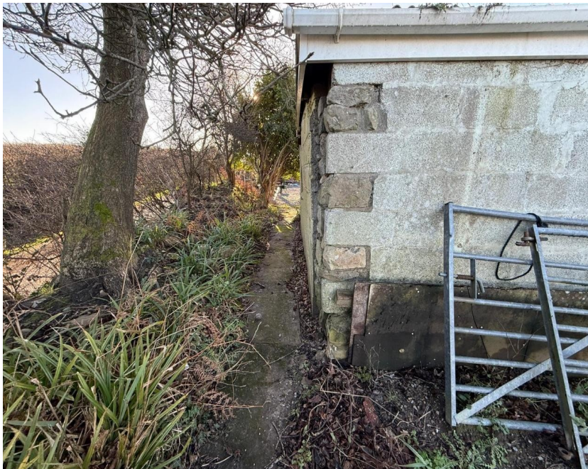
Figure 12: View of garage and proximity to tree / boundary that will be repositioned (moving away from established tree and hedgerow).
