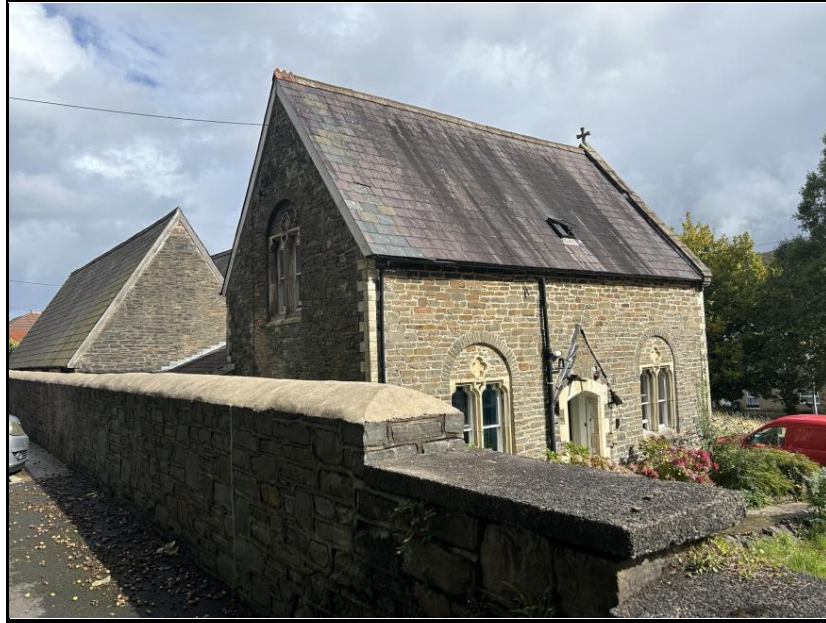
Photograph 3 – Front and Northern Elevations
