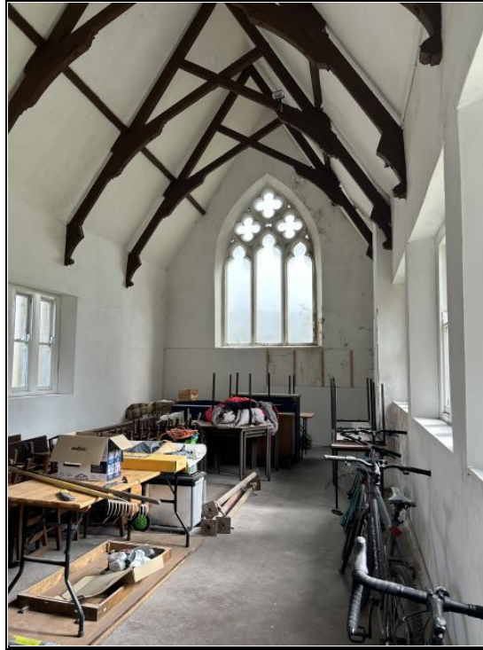
Photograph 11 – Existing Internal Features
