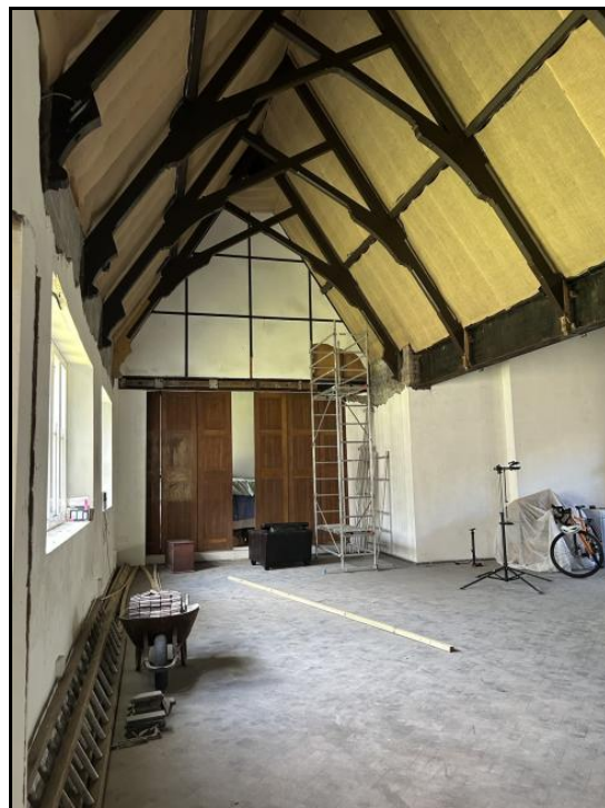
Photograph 10 – Existing Internal Features
