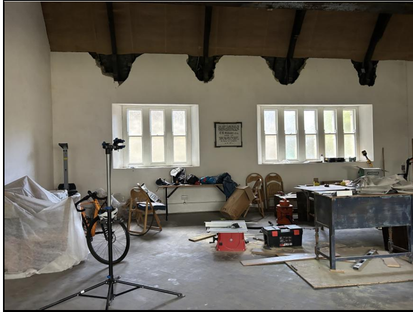
Photograph 9 – Existing Internal Features
