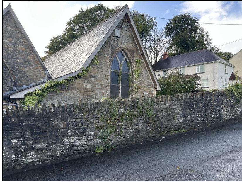
Photograph 5 – Eastern (Rear) Elevation
