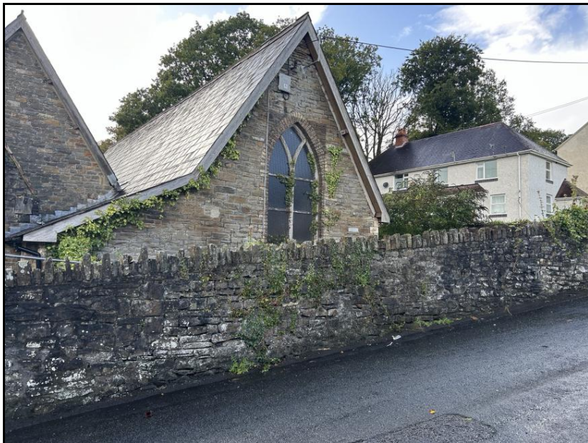
Photograph 5 – Eastern (Rear) Elevation
