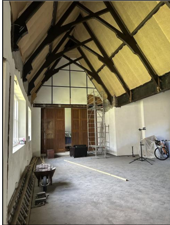
Photograph 10 – Existing Internal Features
