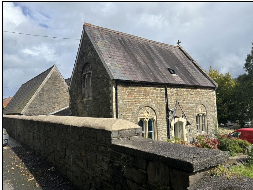
Photograph 3 – Front and Northern Elevations
