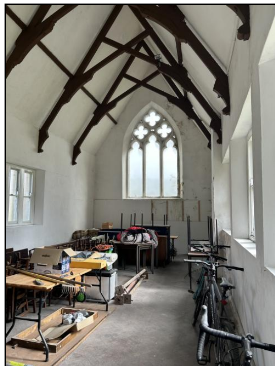
Photograph 11 – Existing Internal Features
