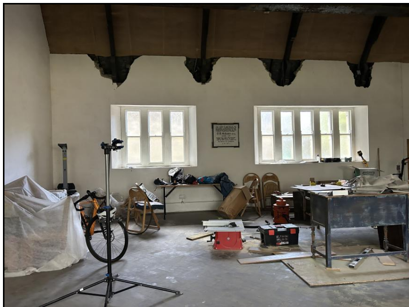
Photograph 9 – Existing Internal Features
