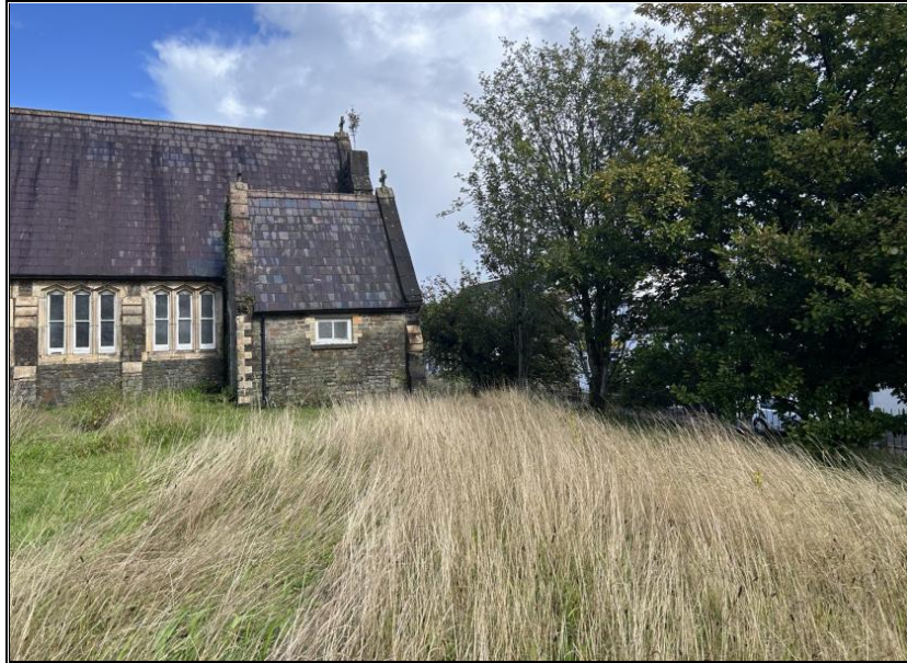
Photograph 8 – Existing Residential Amenity Space
