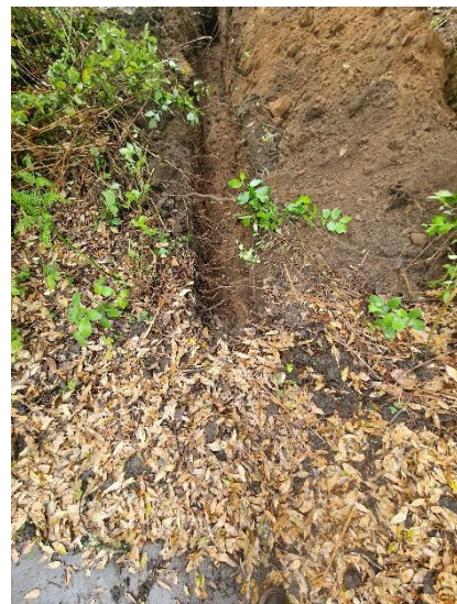
Root in trench toward western end no larger than 1cm in diameter
