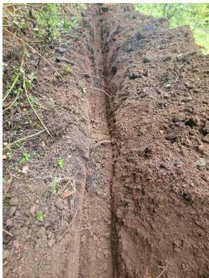
Root in trench toward eastern end no larger than 2cm in diameter
