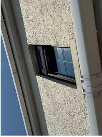
Well-sealed eaves at the hipped roof.
