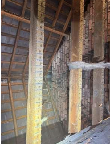
Exposed loft space
