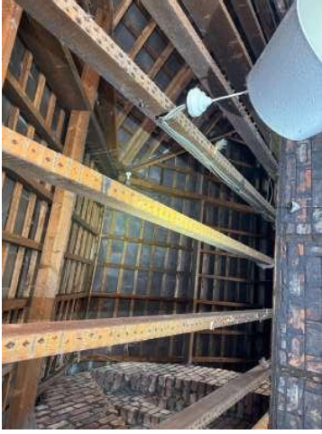
Exposed loft space
