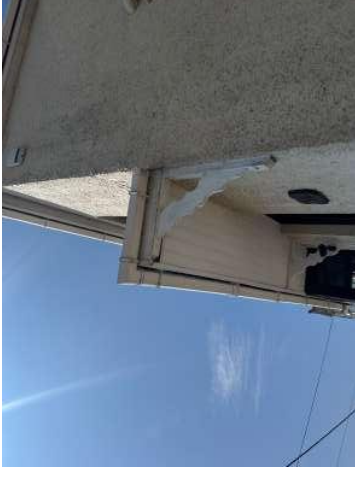
Well-sealed retained soffit box above the porch.
