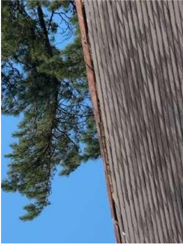
Clay ridge tiles with gaps and well-sealed slate tiles.
