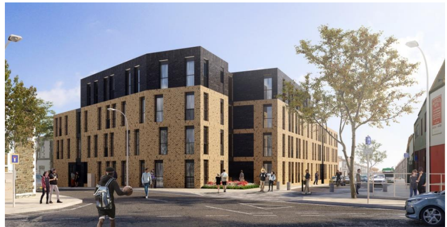
Agate St, Cardiff – Completed scheme for Taff Housing Association
