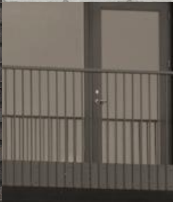
Copper colour Railings (balustrades)
