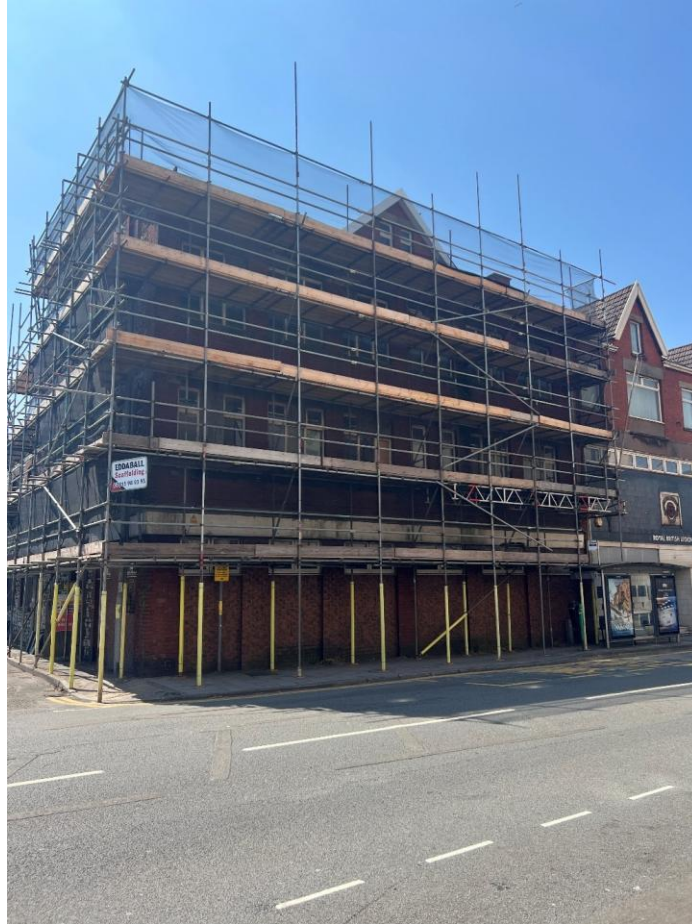
Figure 1.1 Site photograph: existing building frontage onto Talbot Road (July 2026)
