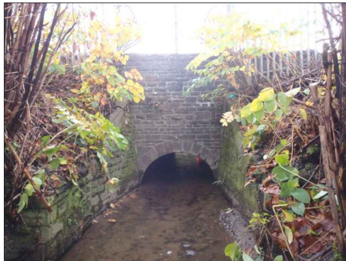
VIEW OF CULVERT ENTRANCE (WEST SIDE)
