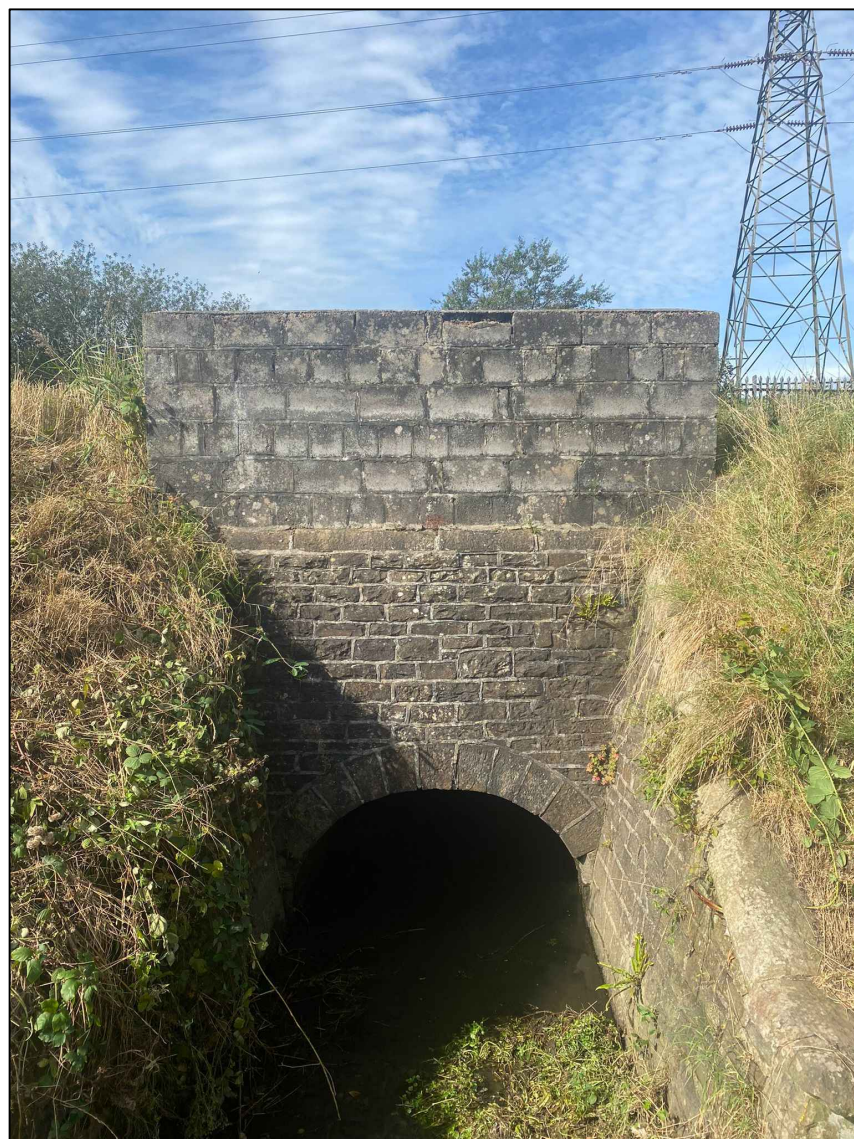
VIEW OF CULVERT ENTRANCE (EAST SIDE)
