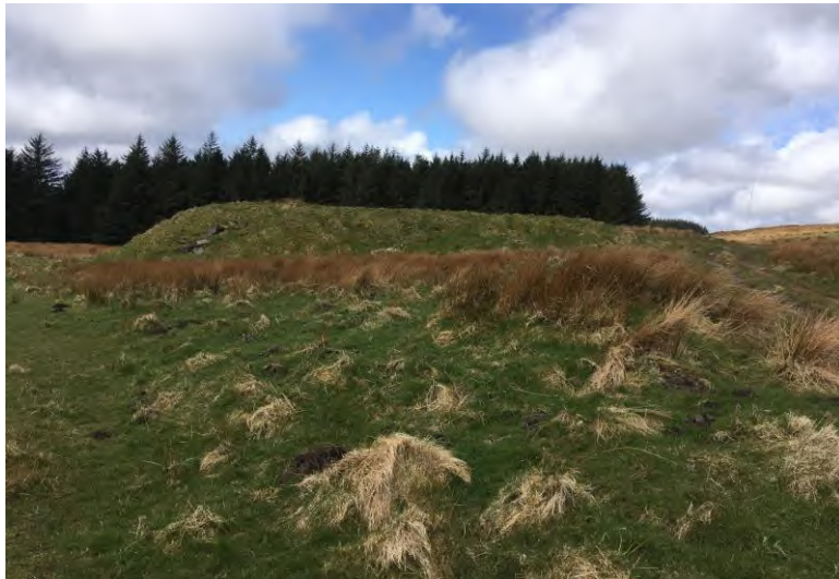
Mound of stockpiled material south of track between T1 and T2.
