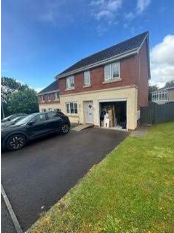
View of front elevation showing existing garage area which is to be converted and tarmac driveway
