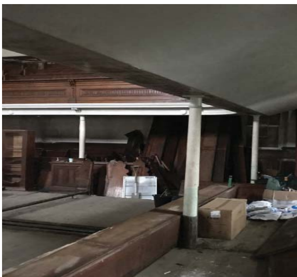
Cast Iron Columns
