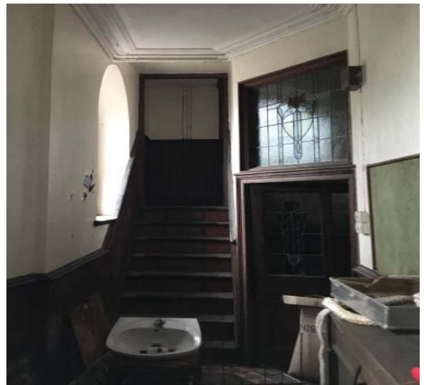
Stair from Entrance Hall 2
