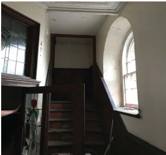
Stair from Entrance Hall 1
