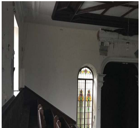
First Floor Raked Seating and Full Height Stained Glass Window
