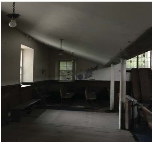
Underside of Raked Seating Area
