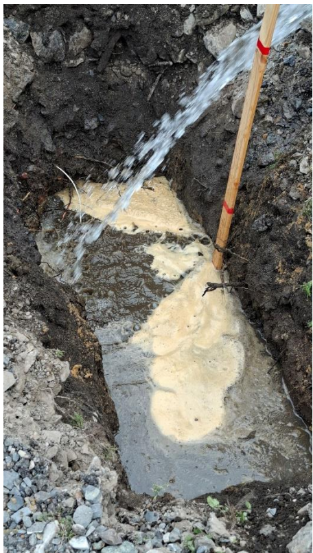
Figure 7 - Test hole filling
