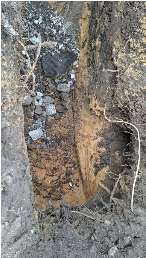
Figure 3- Test hole excavation
