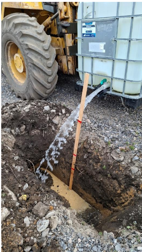
Figure 6 - Test hole filling
