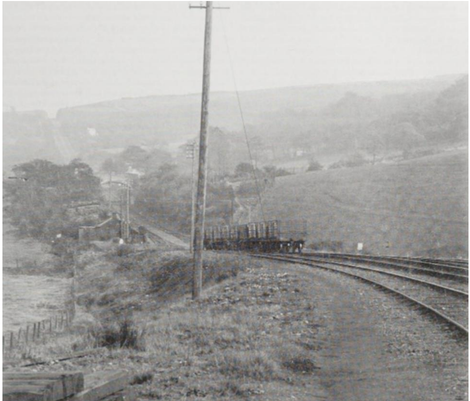
Figure 5-3 - Historic image dating from the early 20th century showing the base of the Incline looking east. The structure visible to the left of the line is likely to represent the structure visible on historic Ordnance Survey maps close to the modern entrance to the playpark. Reproduced from Simmonds 2012, A History of the Port Talbot Railway & Docks Company and the South Wales Mineral Railway Company. Volume 1: 1853 – 1907.
