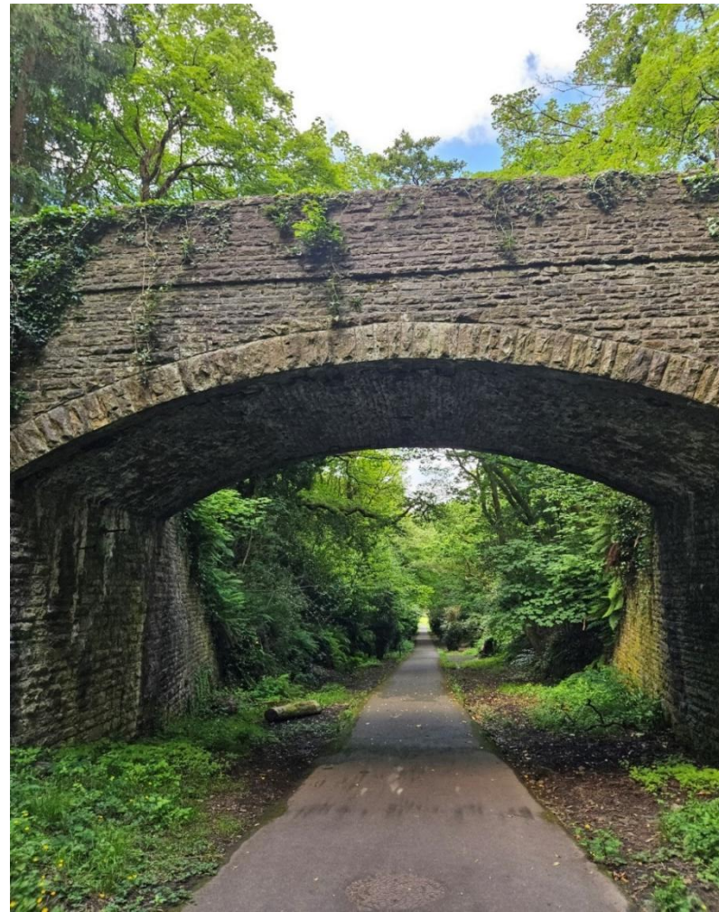
Figure 5-5 - Bridge over Ynysmaerdy Incline (23308)
