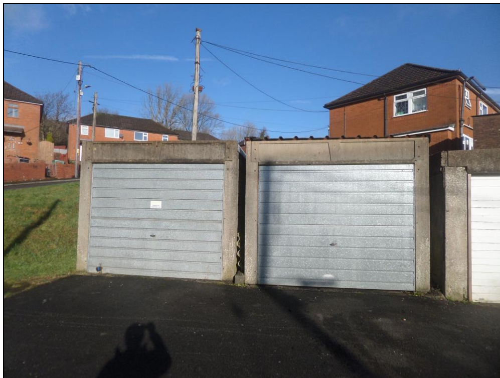
Photo 3: Garages 1 & 2 (west to east) (view looking north).
