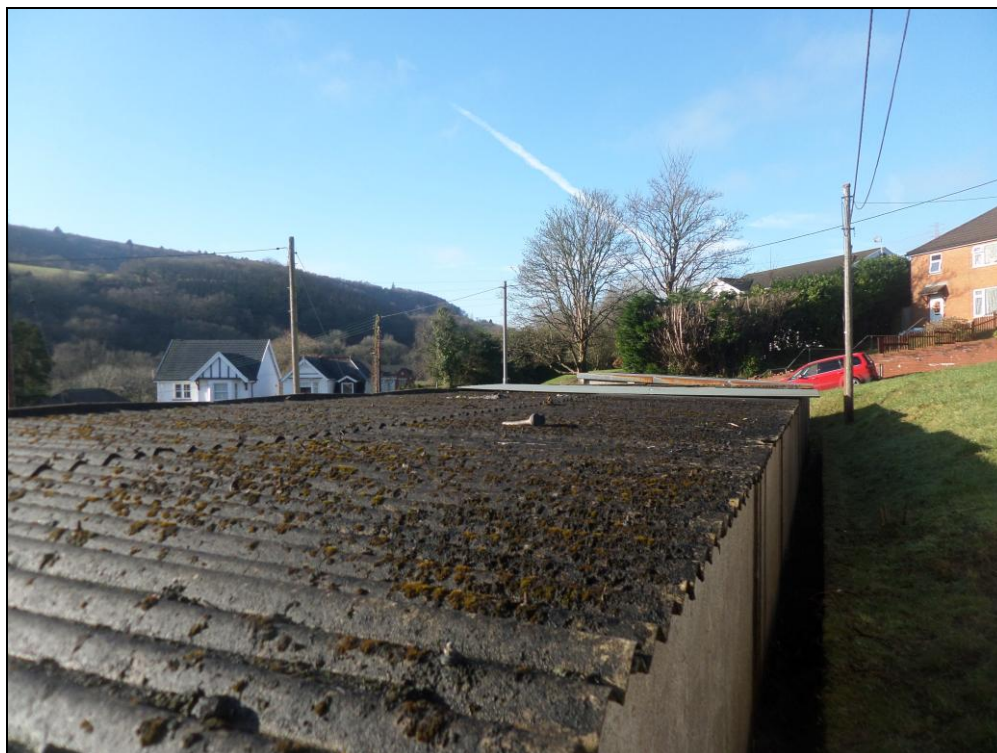
Photo 6: Corrugated asbestos and metal flat roof on garages (view looking west).
