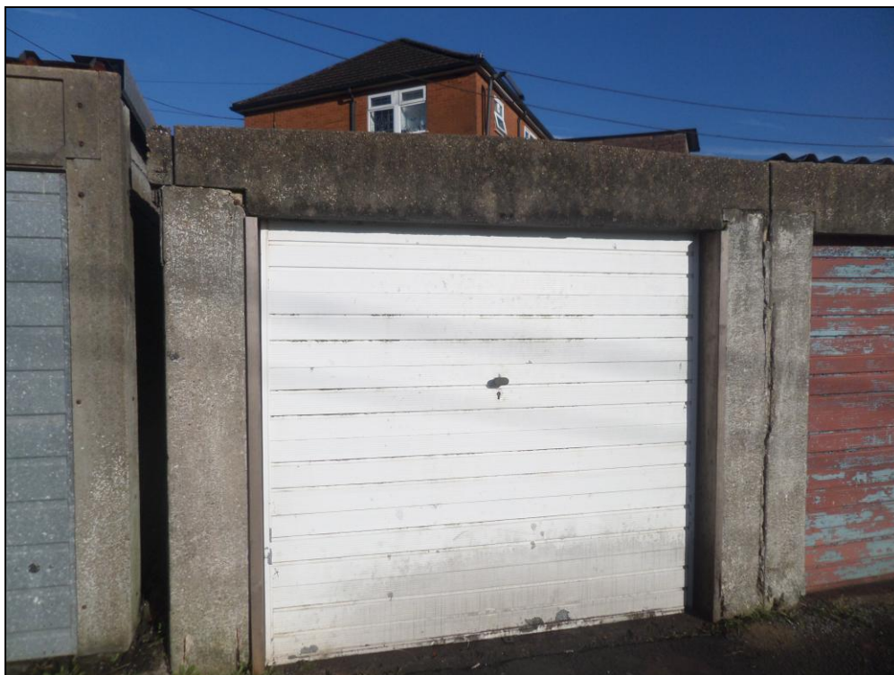
Photo 4: Third garage (west to east) (View looking north west).
