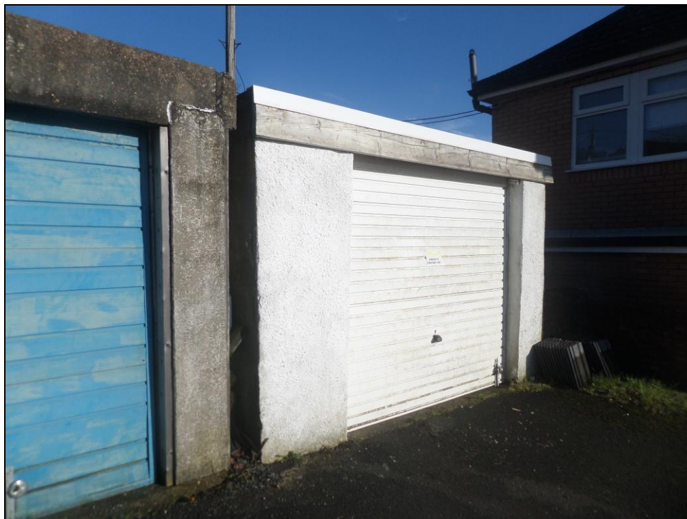
Photo 7: Detached garage 9 (View looking north east).
