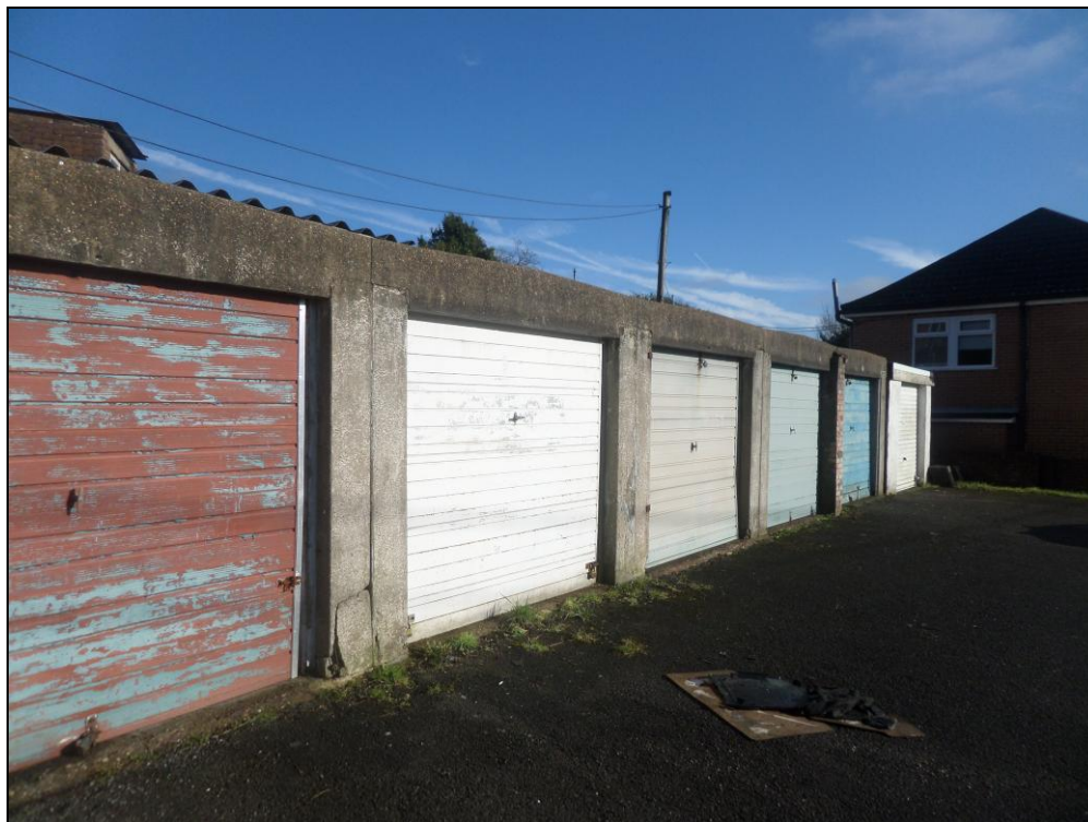
Photo 5: Garages 4 – 9 (west to east)(view looking east).
