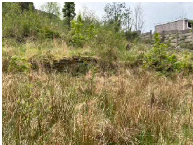
View of stone walling
