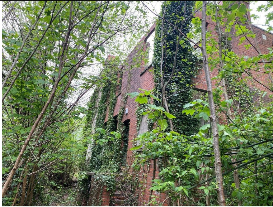
Plate 3: Southern and eastern elevation of main house
