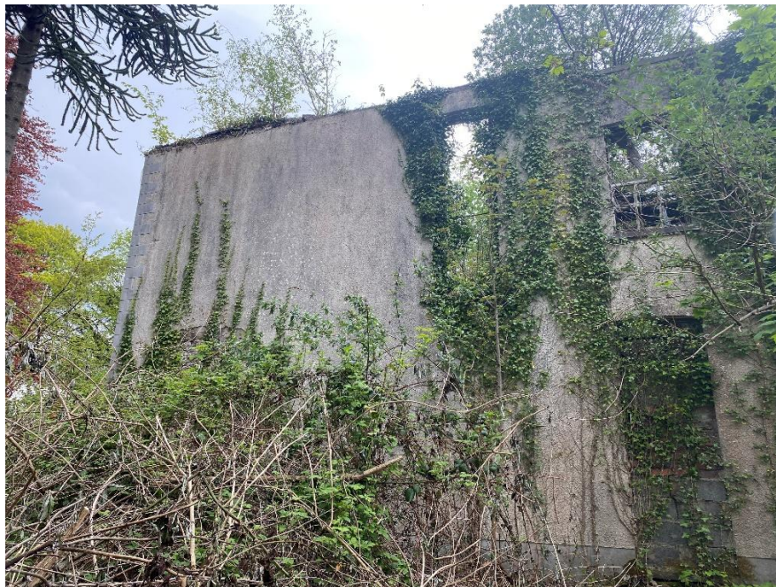
Plate 2: Western elevation of main house
