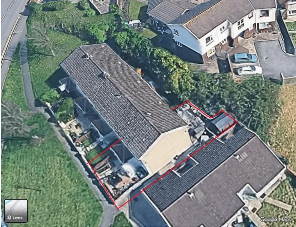
Site context view showing application site edged red and adjacent boundary vegetation.
