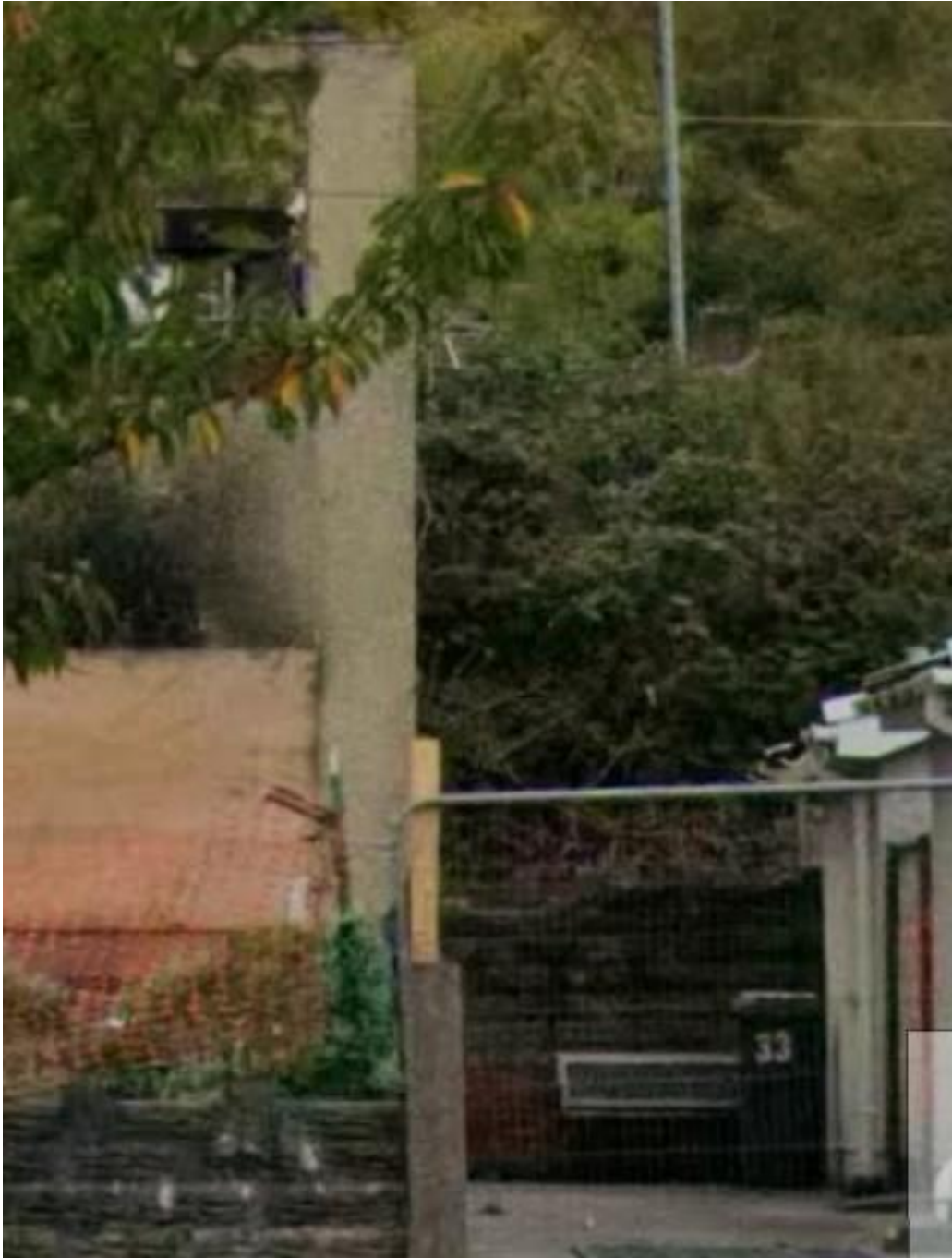
Figure 3: Street view image showing the existing frontage to No. 33 and boundary vegetation visible beyond/adjacent to the site. The vegetation comprises dense bushes, scrub and self-seeded growth and is to be retained.
