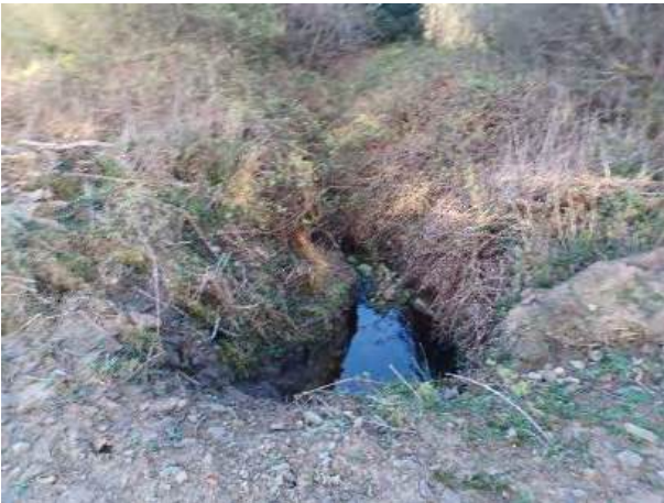
08.04.26 – View of culverted stream beneath access track
