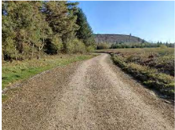
08.04.26 – View north up the access track
