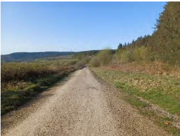
08.04.26 – View back south down the access track
