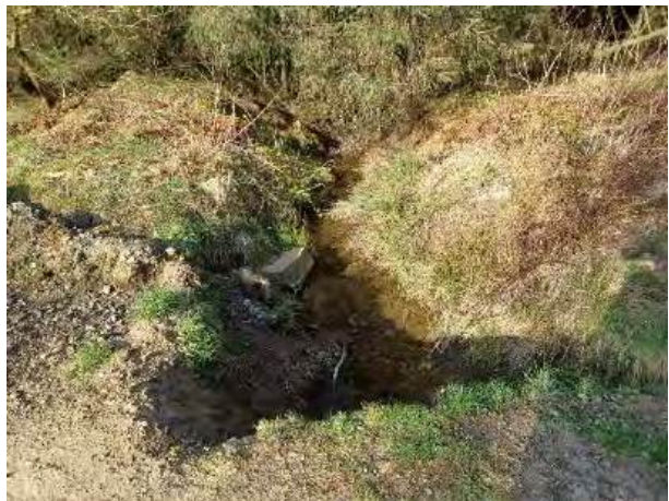
08.04.26 – Stream culverted beneath access track
