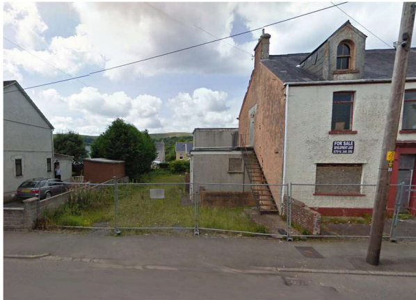
Existing Access into Site (to be retained)
