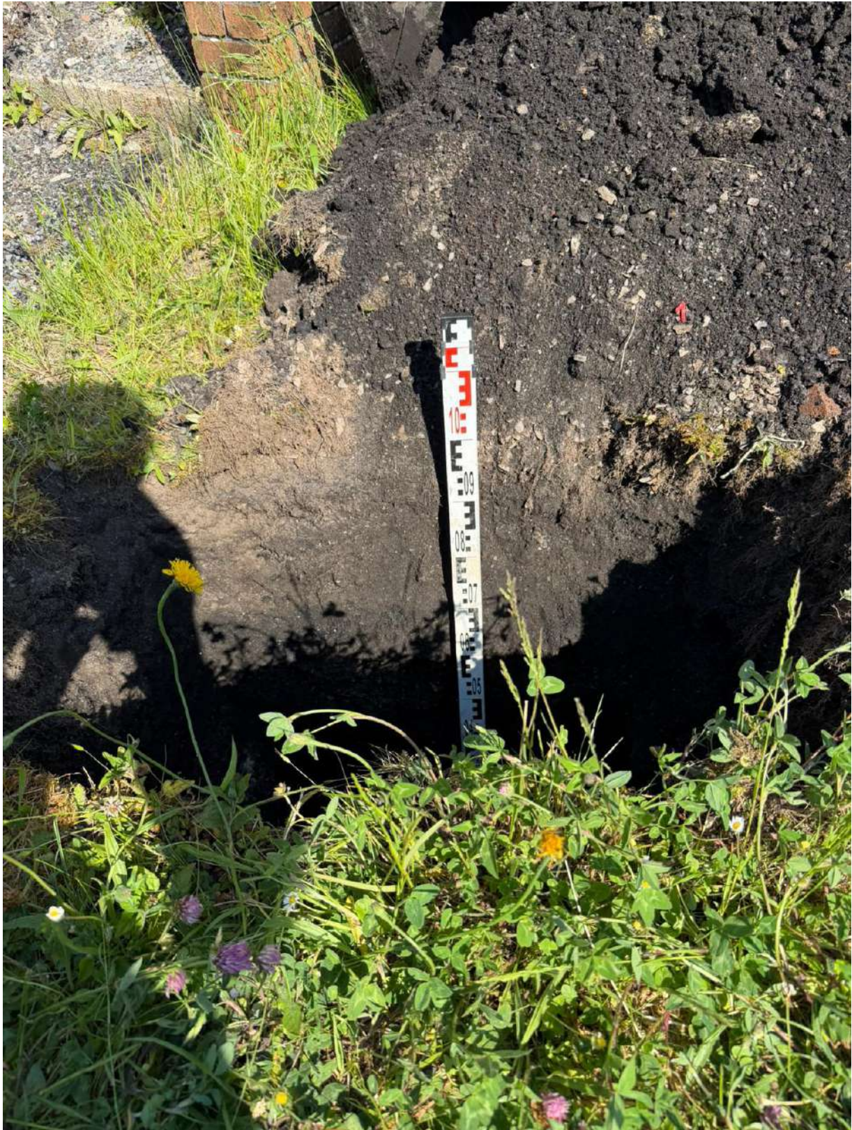
Figure 2 - Test pit 1 during excavation
