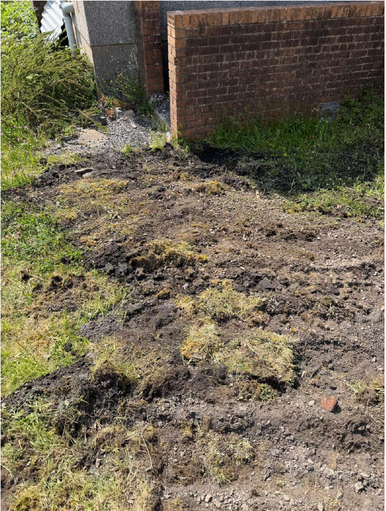
Figure 8 - Test pit remediation
