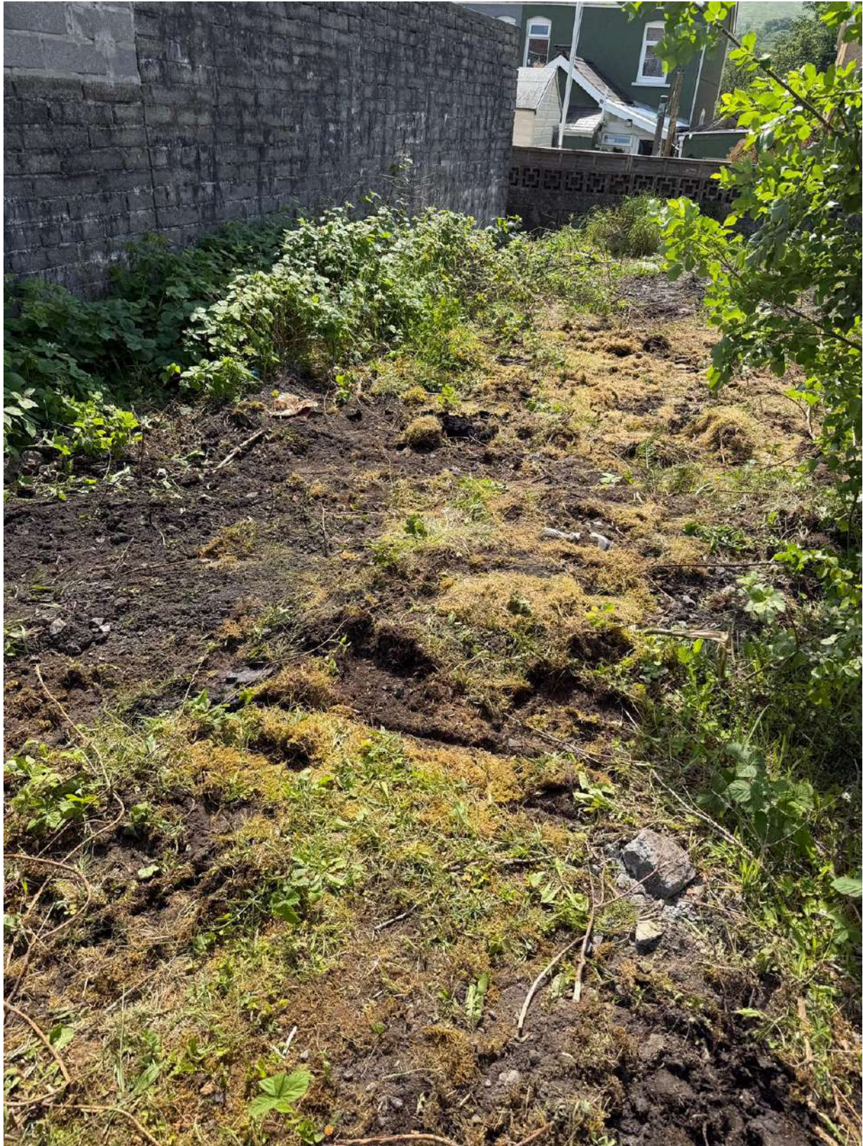
Figure 9 - Test pit remediation
