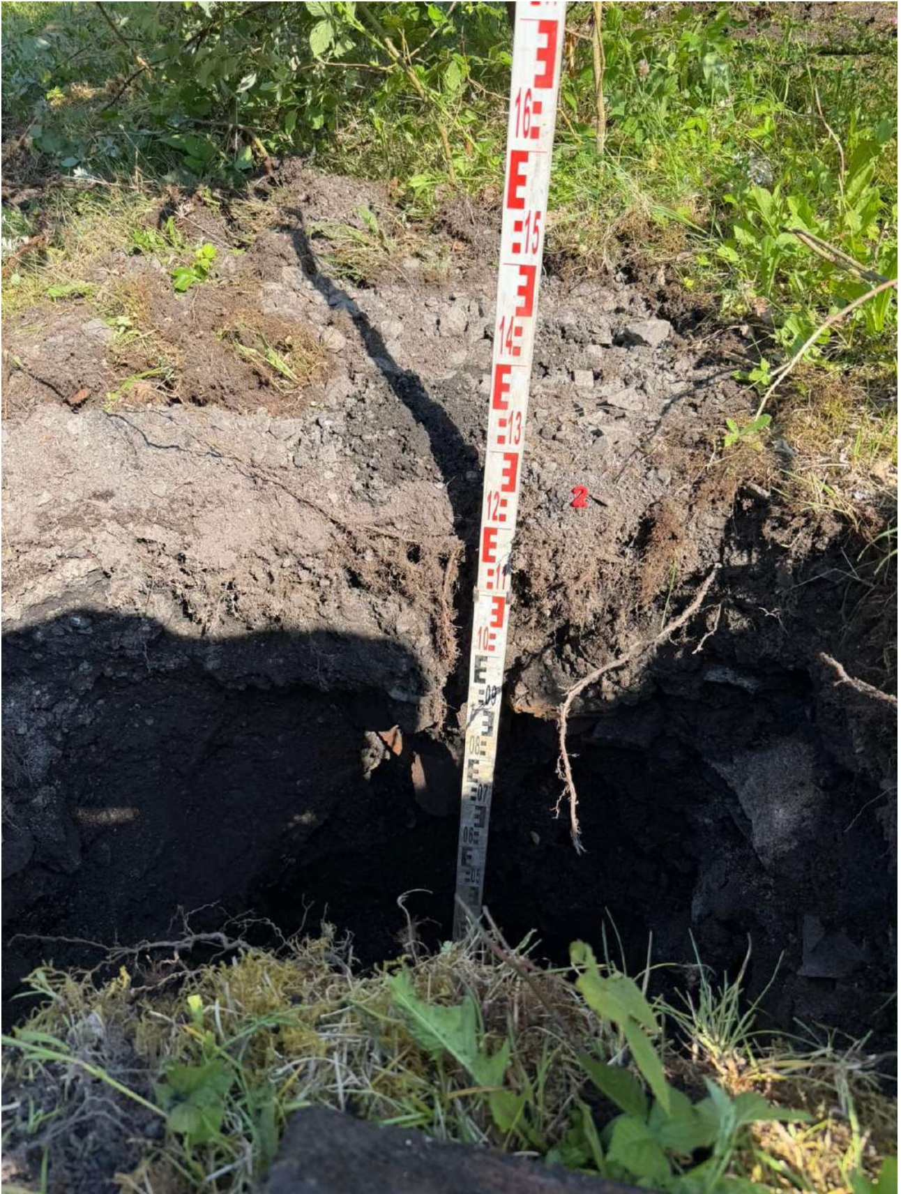
Figure 5 – Test pit 2 during excavation
