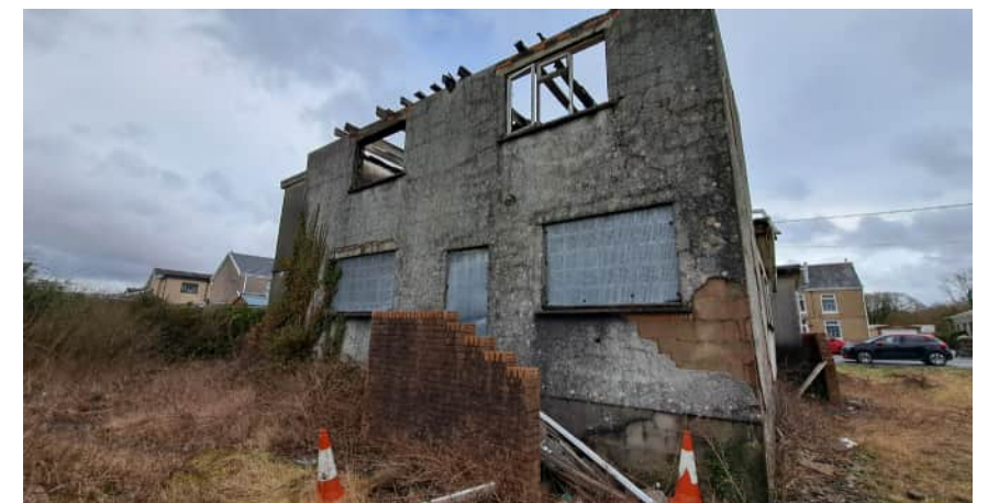
Northern boundary with overgrowth of mixed planting
