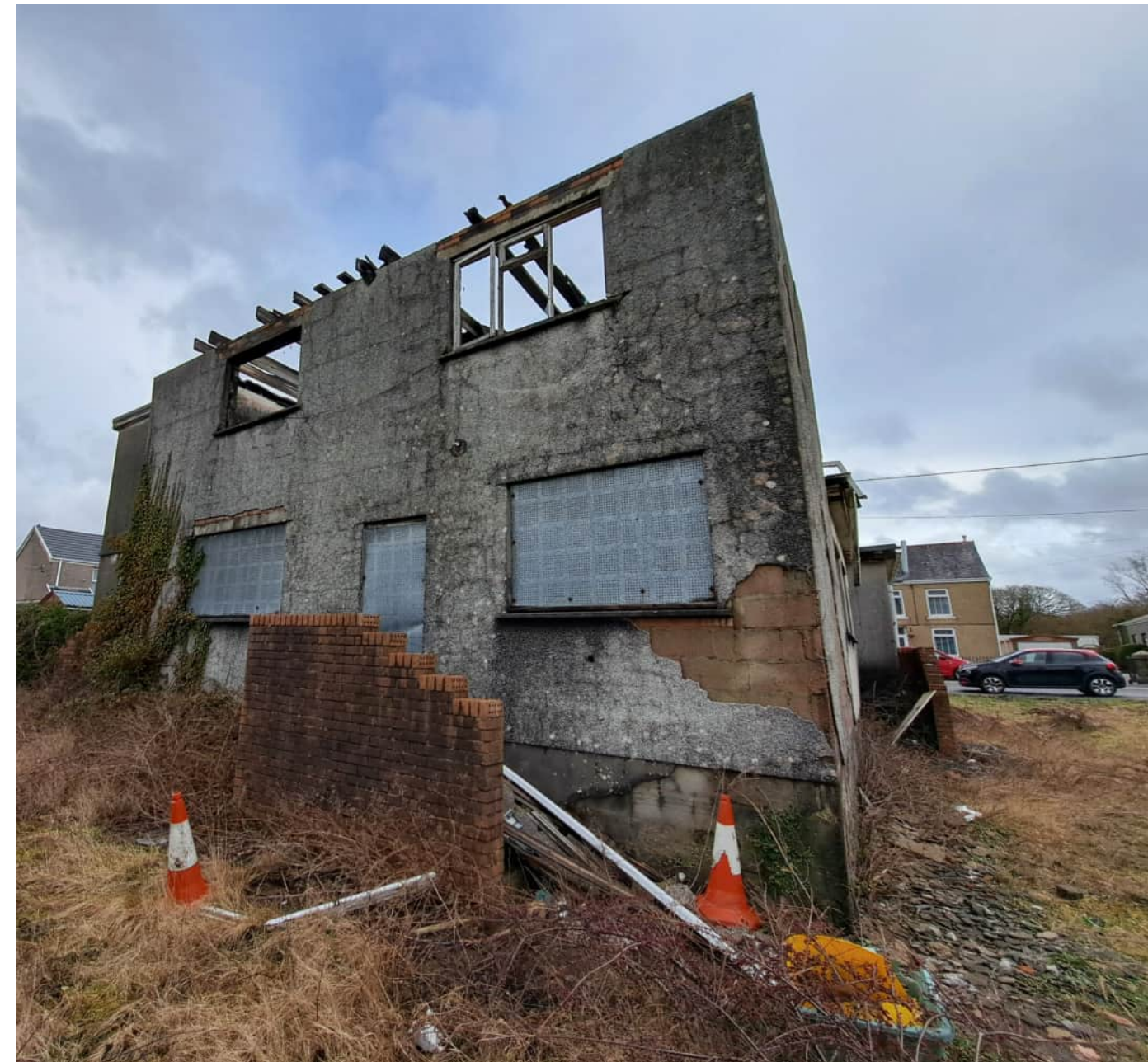
View of the site seen from the south west. Vehicular access entry point is visible to the right of the building.
