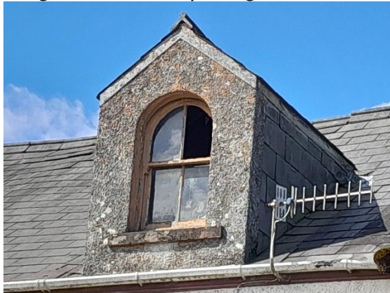
Image 2: Window opening in dormer
