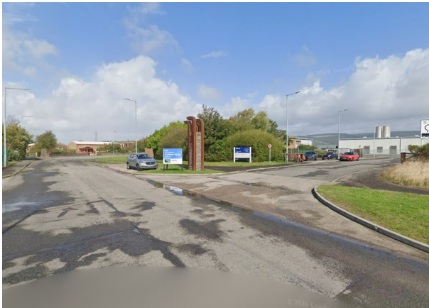
Road width of the industrial estate is wider to suit the large vehicles used for delivery.
