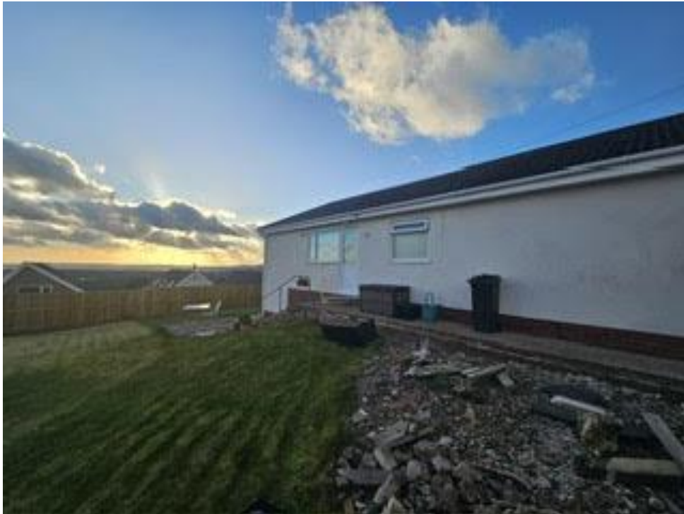
Side elevation view where the new balcony area will be sited
