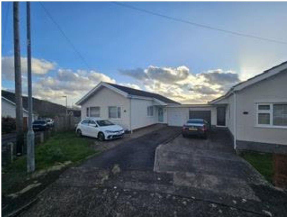
View of front elevation showing existing tarmac driveway and small lawn area
