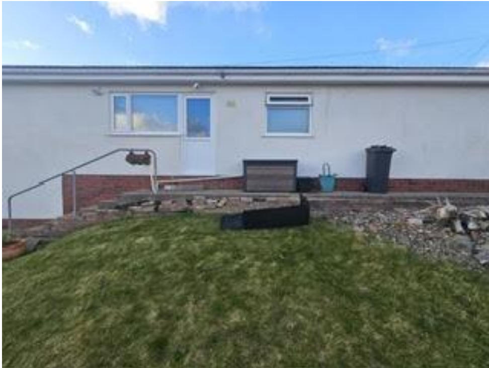
View of side elevation where the new decking area will be sited.
