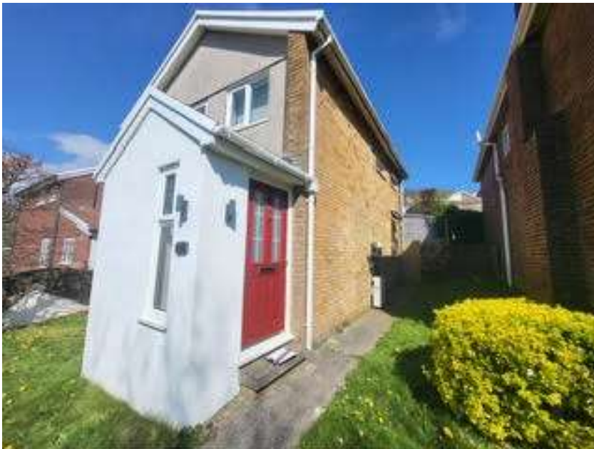
Front and side elevation view concrete path leading to rear garden area and small lawn to side
