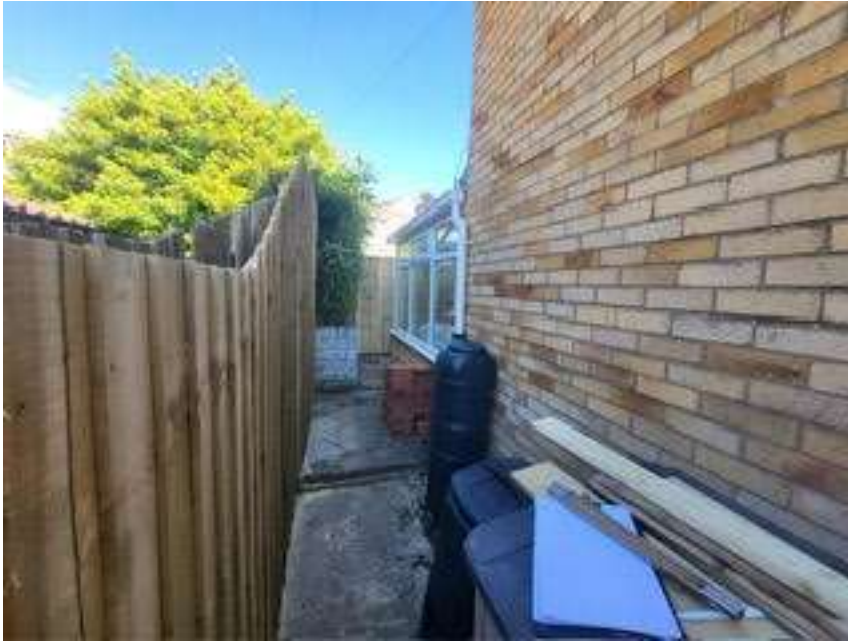
View of side elevation where the new side extension will be sited. Timber fence panels already in place
