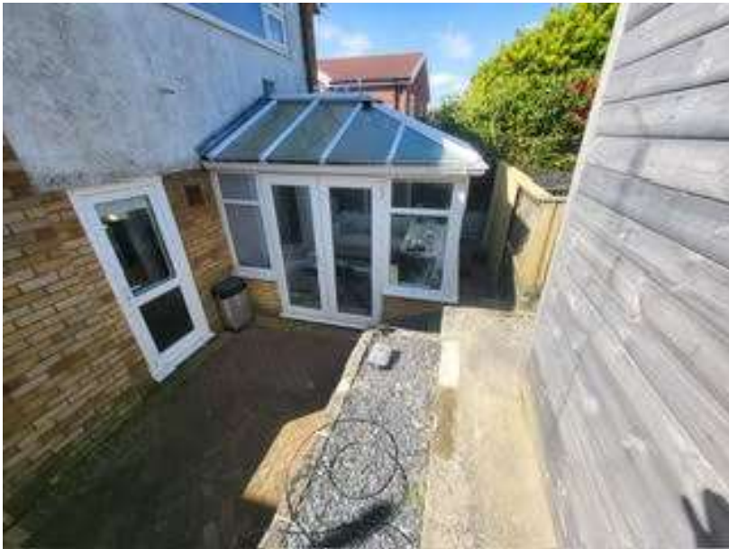
Existing rear conservatory where the new two storey extension will be sited.
