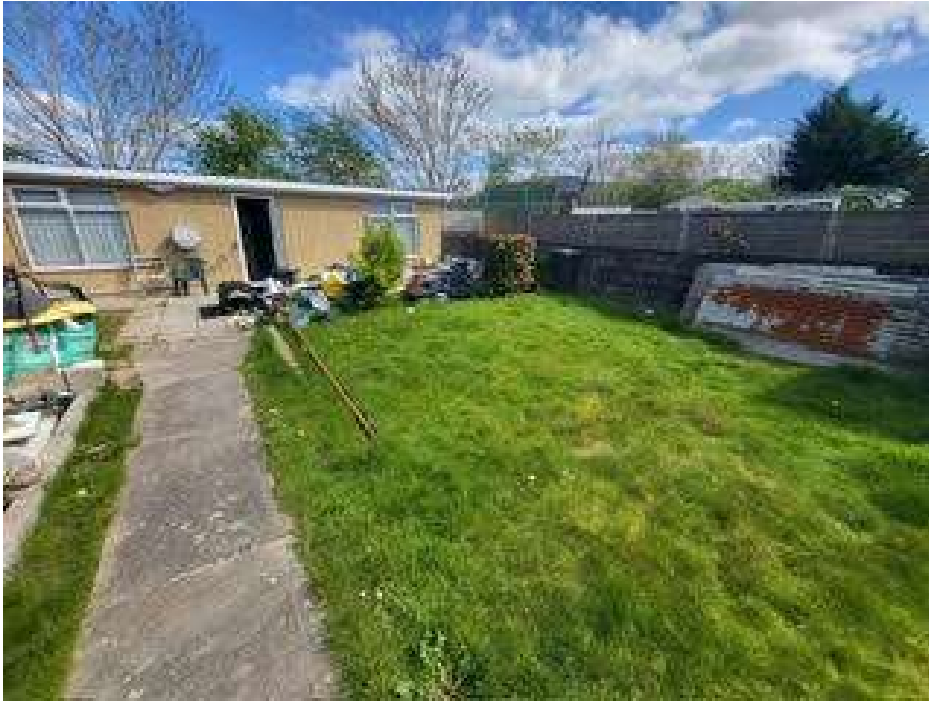
Further view of rear elevation showing existing outbuilding and large lawned garden
