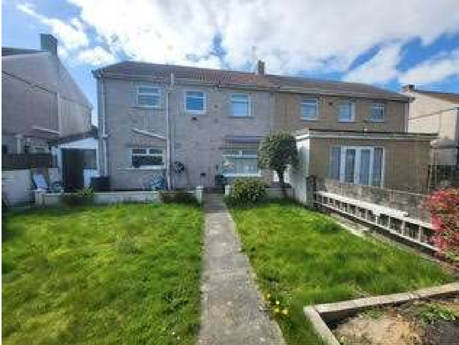
Rear elevation view where the new rear extension will be sited. Neighbours existing extension can be seen. Existing lean to extension can also be seen, this is to be removed.
