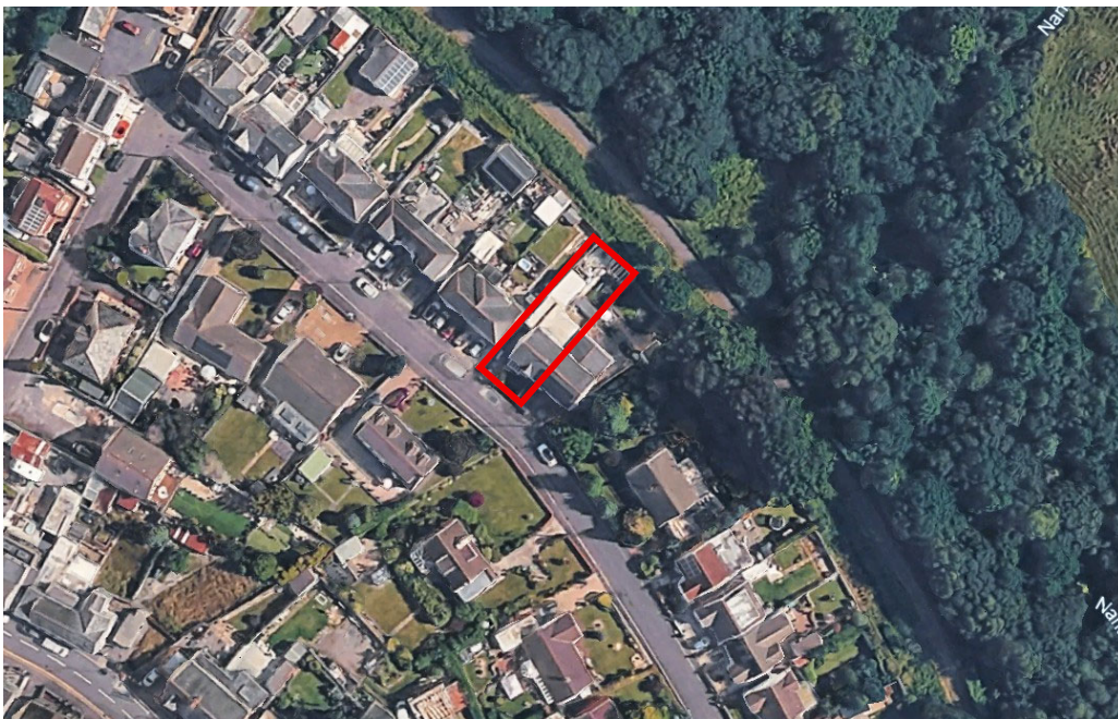
Enlarged view of application site
