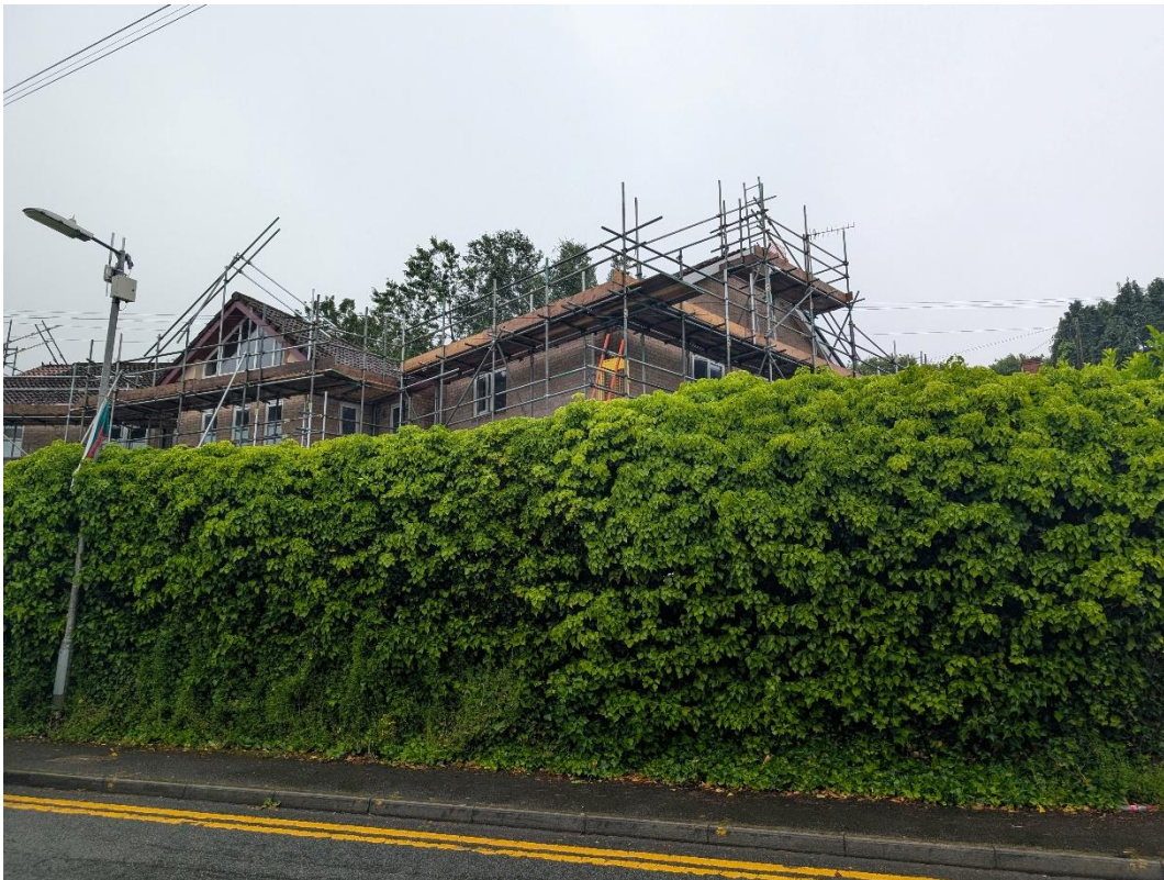
Existing hedgerow which forms a strong green boundary feature to the front of the site to be retained and maintained
