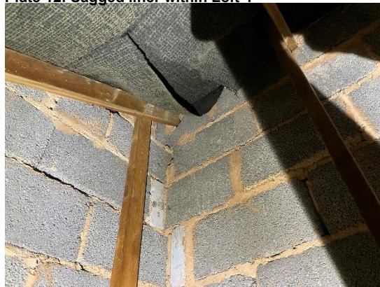
Plate 12: Sagged liner within Loft 4
