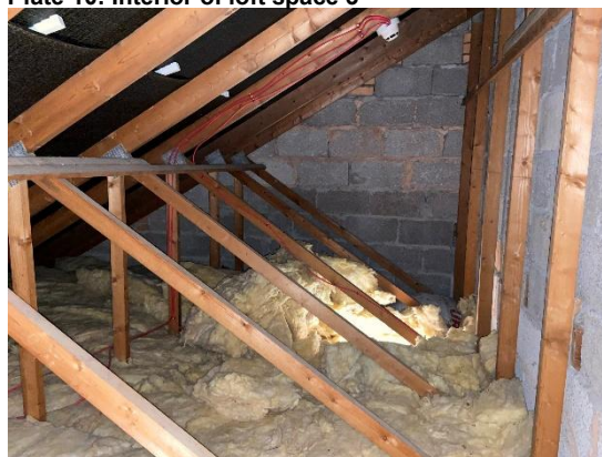
Plate 12: Sagged liner within Loft 4
