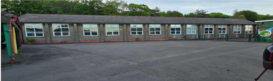
South elevation of the school showing slate roof
