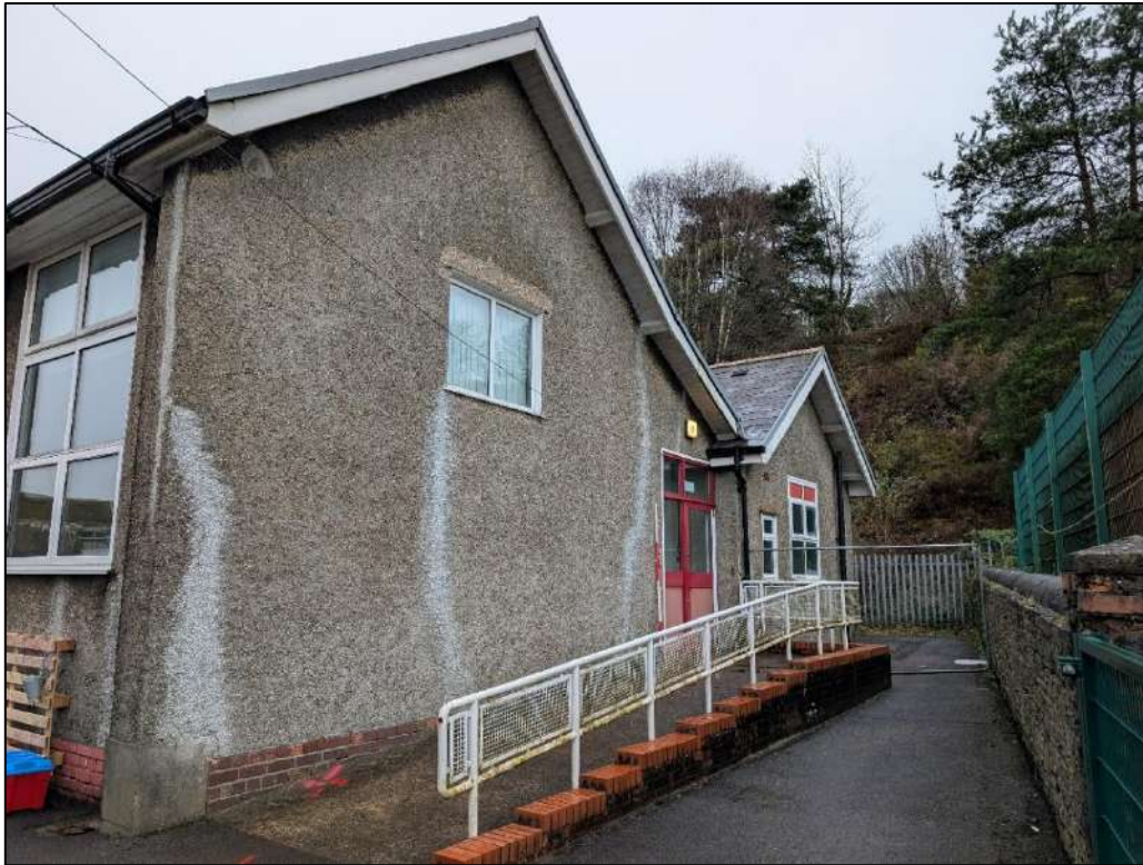
Plate 3. East facing elevation, view to the north-west.
