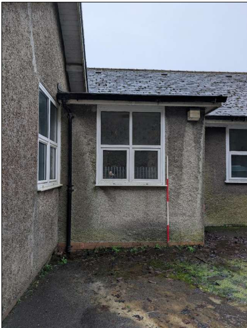
Plate 13. Northern elevation of eastern square extension, view to the south.
