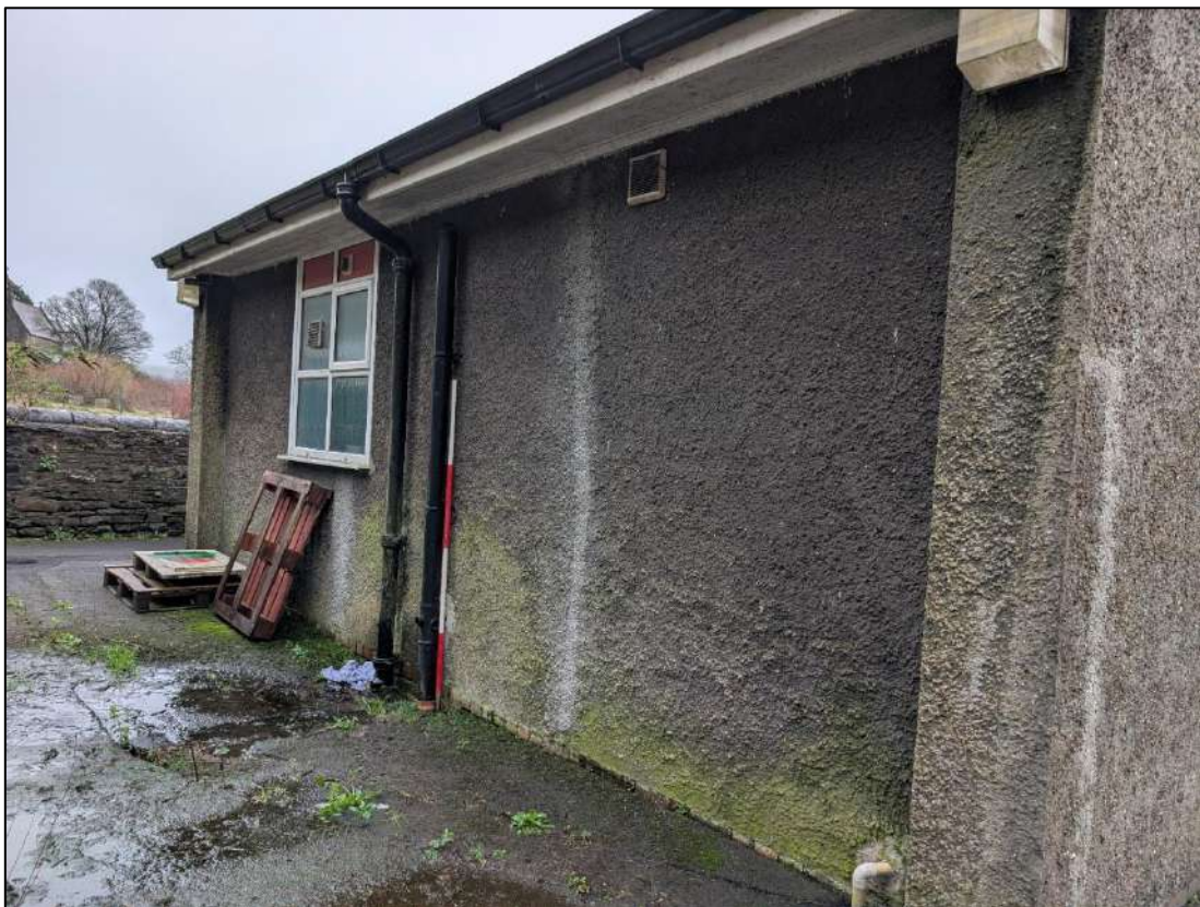
Plate 10. North facing elevation of eastern range, view to the south-east.
