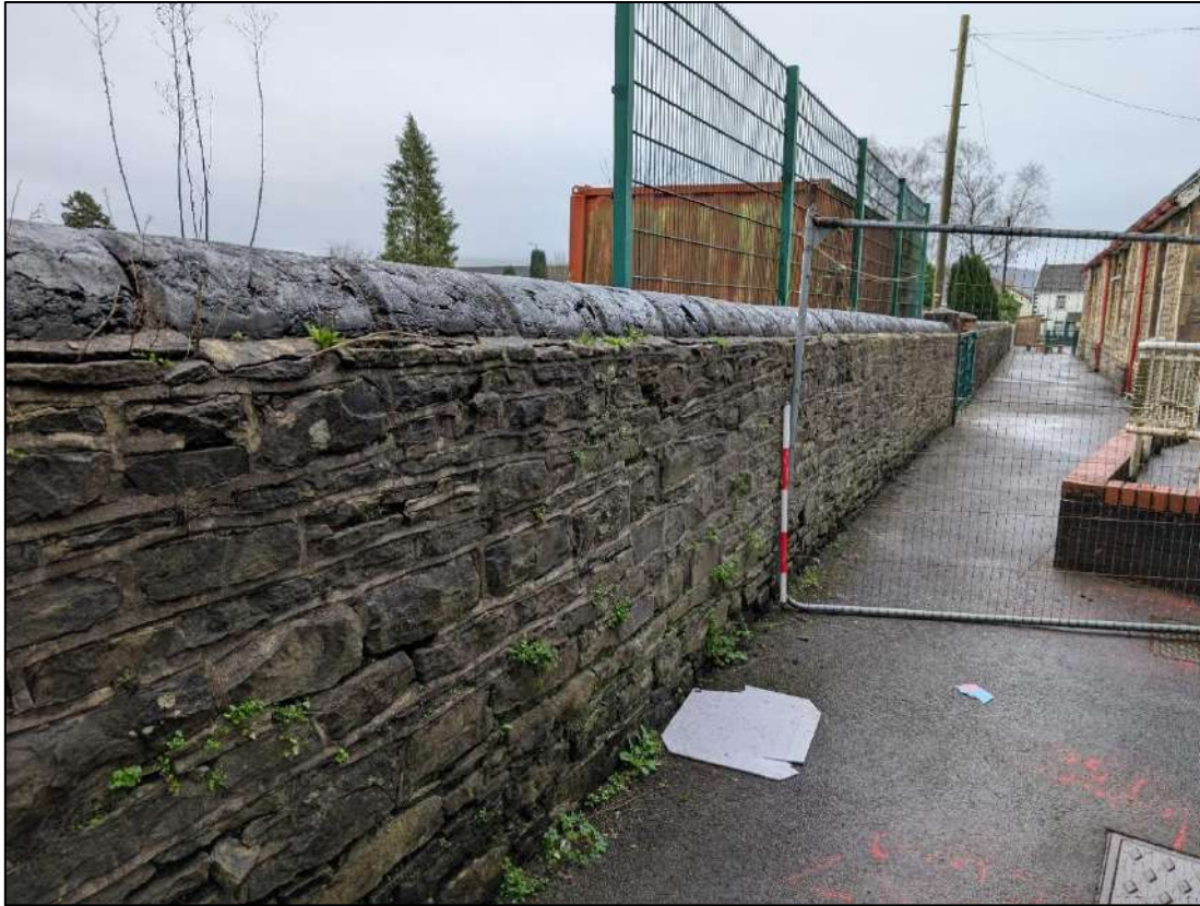
Plate 45. West facing elevation of boundary wall, view to the south-east.
