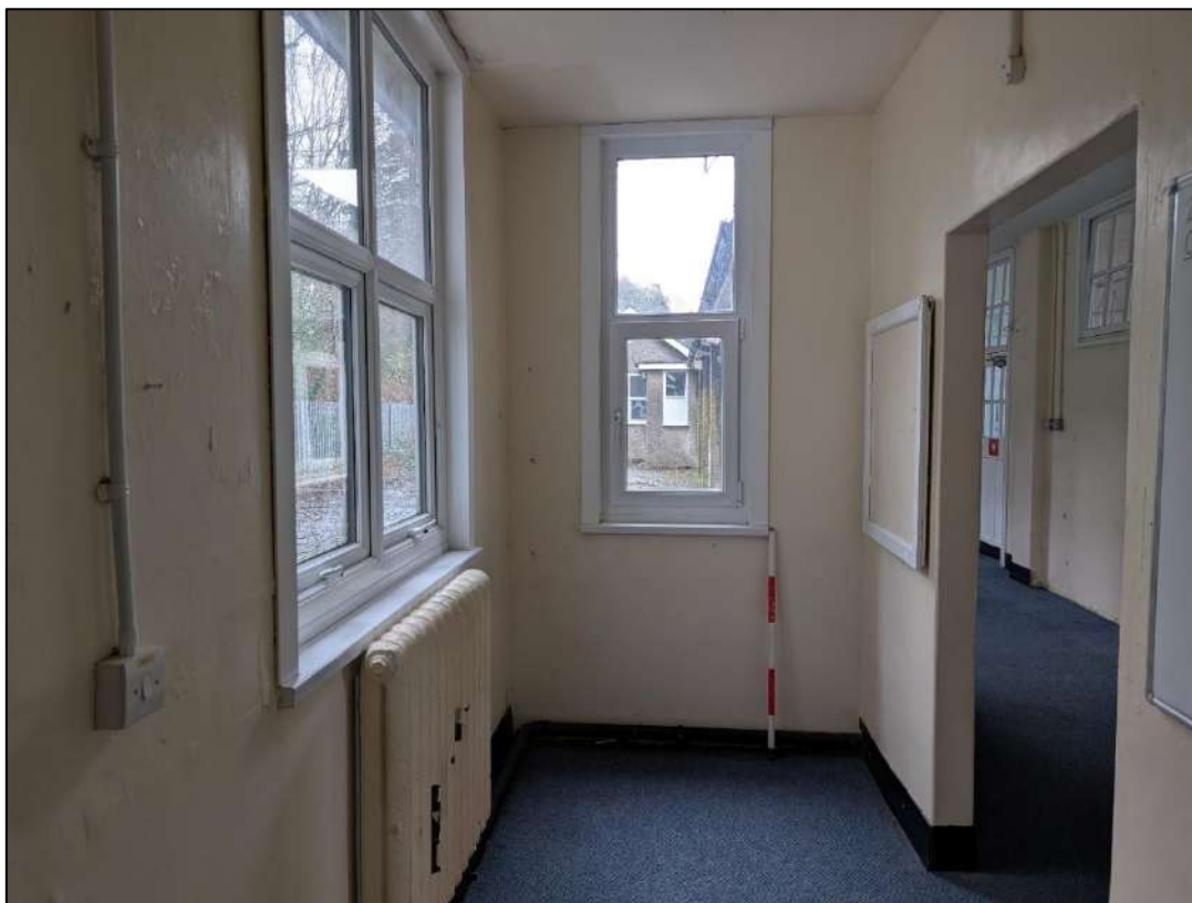
Plate 38. Room 13 view to the east.
