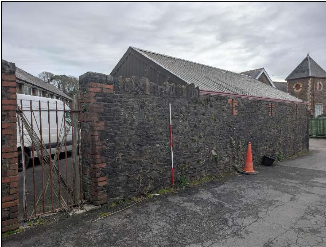
Plate 49. Western elevation of boundary/shed wall, view to the south-east.
