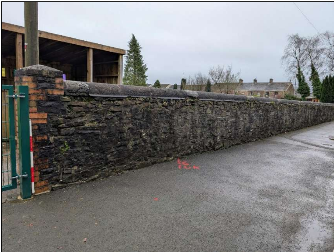
Plate 46. West facing elevation of boundary wall, view to the south-east.
