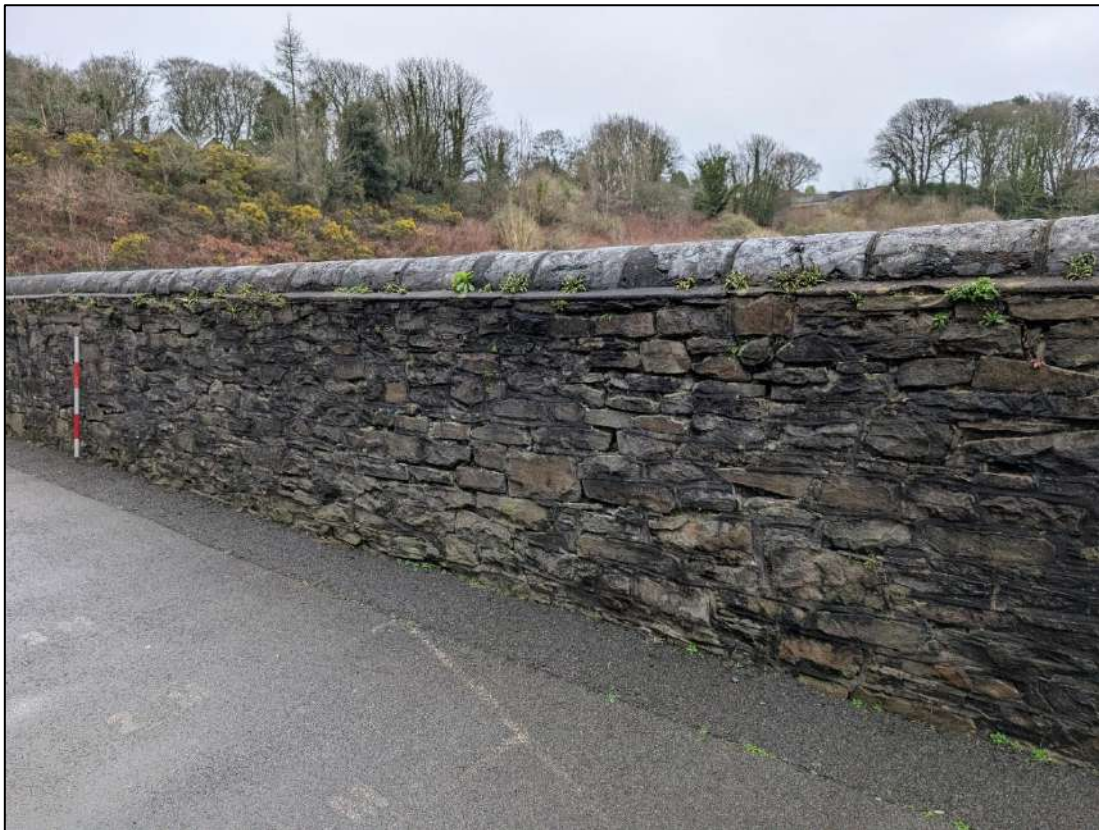
Plate 44. West facing elevation of boundary wall, view to the north-east.
