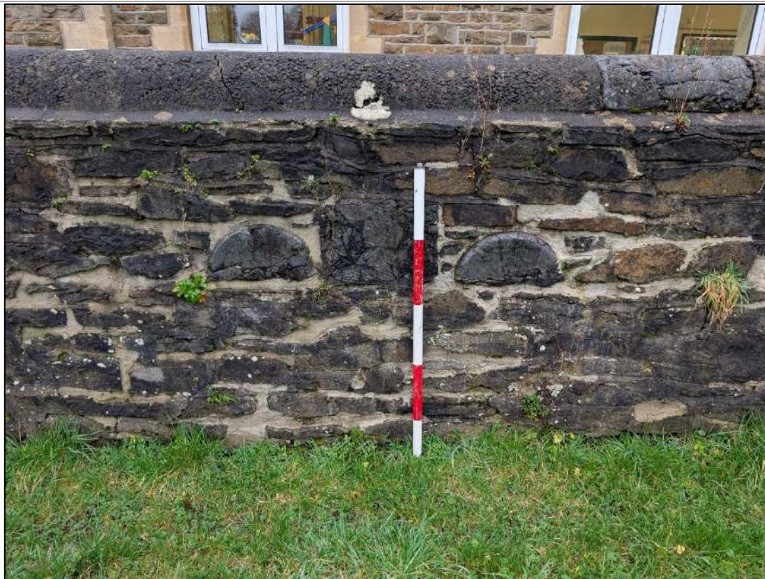
Plate 47. Eastern side of boundary wall showing the slag used within construction, view to the west.
