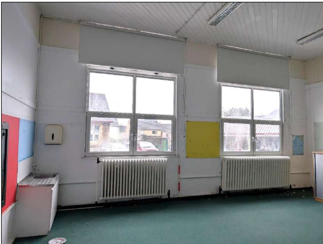
Plate 18. Southern wall of classrooms, view to the south-west.
