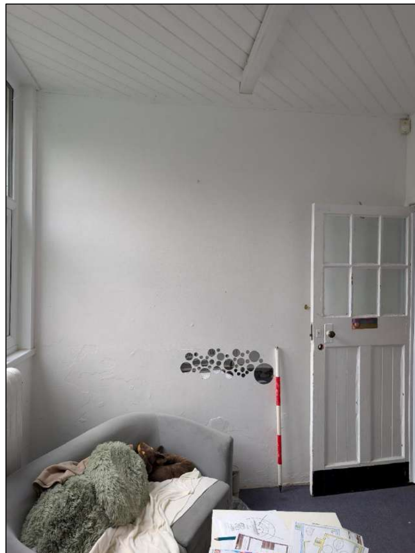
Plate 40. Room 14, view to the south-west.
