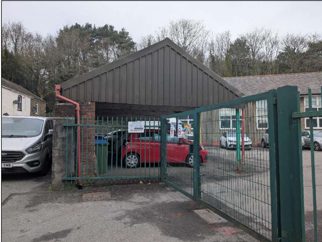
Plate 53. Corrugated sheeting used within shed building and exiting gateway, view to the north.
