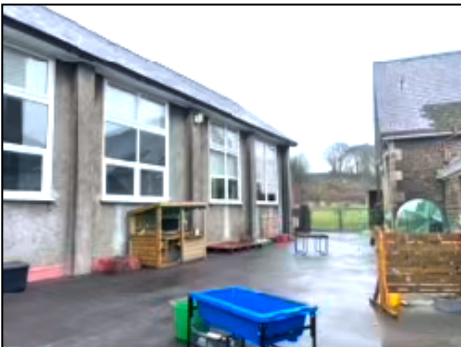
Photo 11. Hardstanding area within centre of school buildings and entrance gate into eastern field.
