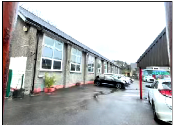
Photo 12. Central hardstanding parking area within school buildings.
