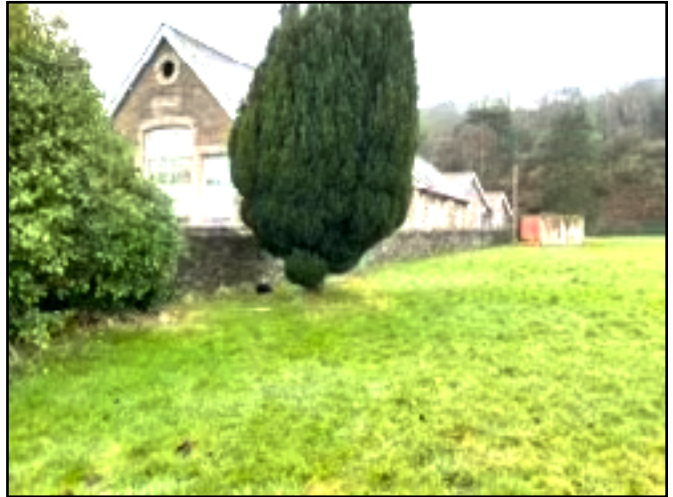
Photo 2. Western wall between field and school buildings.
