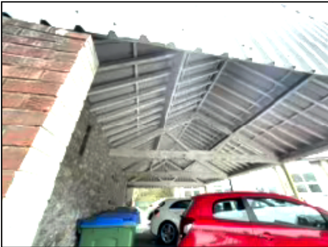
Photo 9. Car shelter structure roofing.
