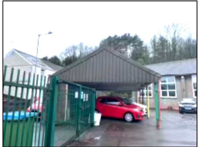
Photo 8. School grounds with metal car shelter structure in west of site.
