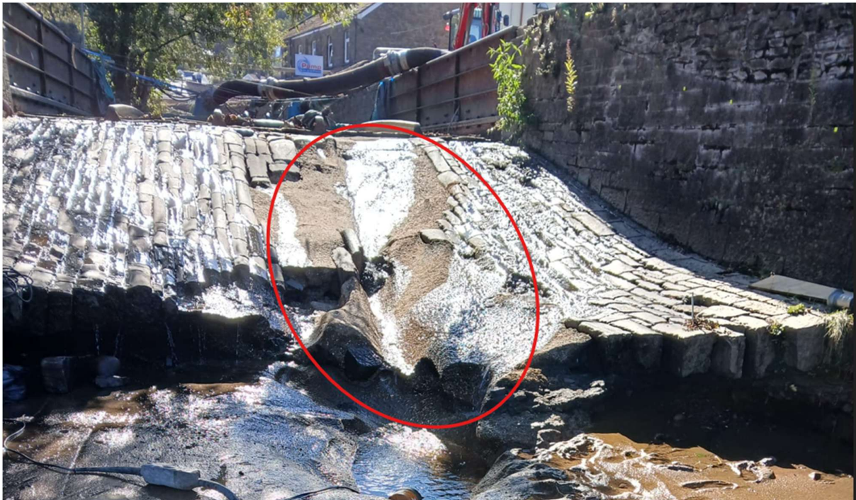
Figure 1 existing concrete to be broken up and removed
