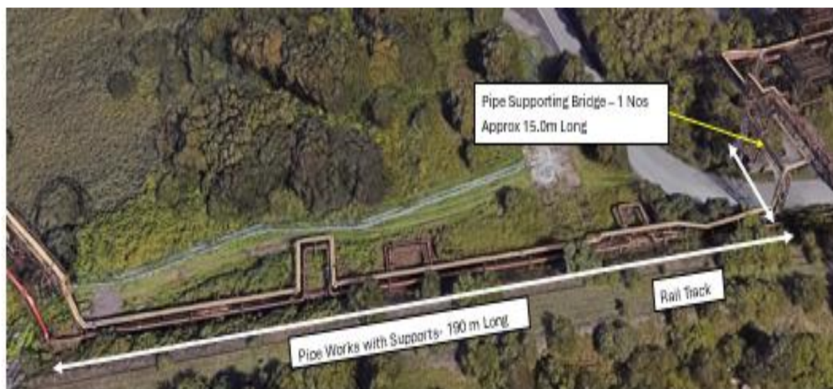
Fig. 5 Pipework Including Support Bridge
