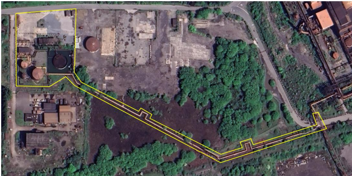
Fig -1: Overview of Phoenix Oil Tank Farm
