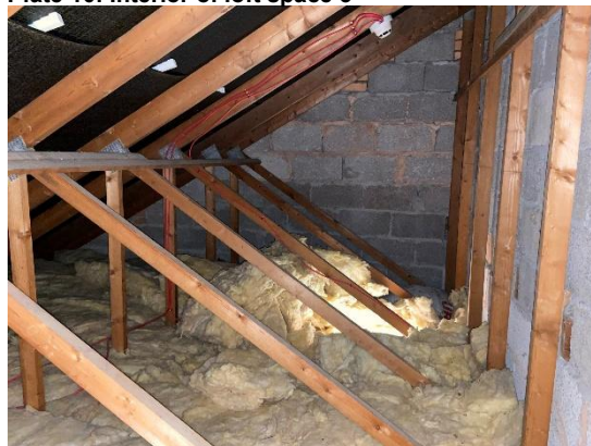
Plate 12: Sagged liner within Loft 4
