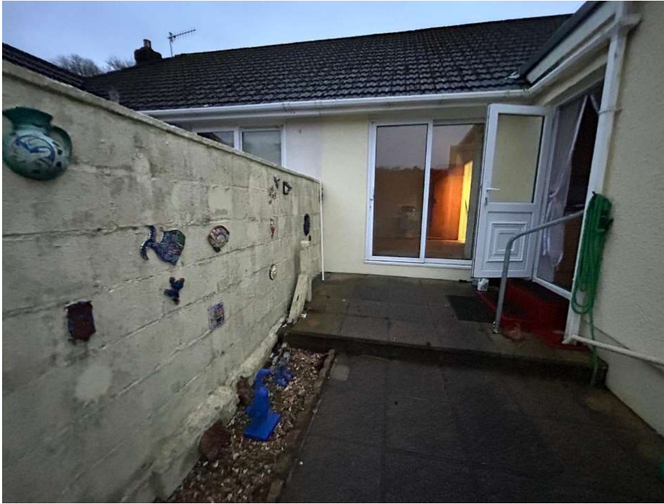
View of area where new extension will be made wider
