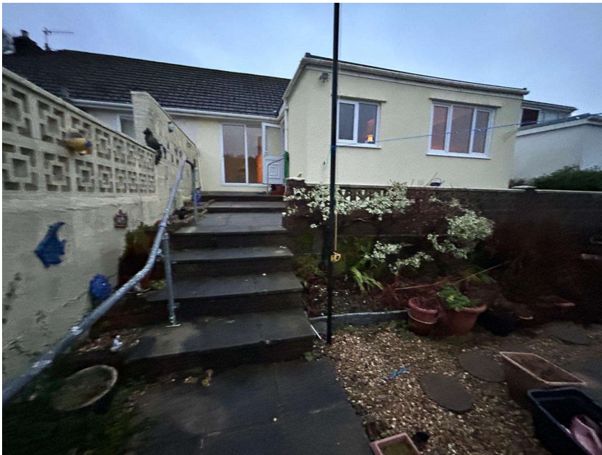
View of rear elevation and area where new extension will be made slightly wider. This area is currently a hard surfaced patio area. Steps to lower garden can be seen
