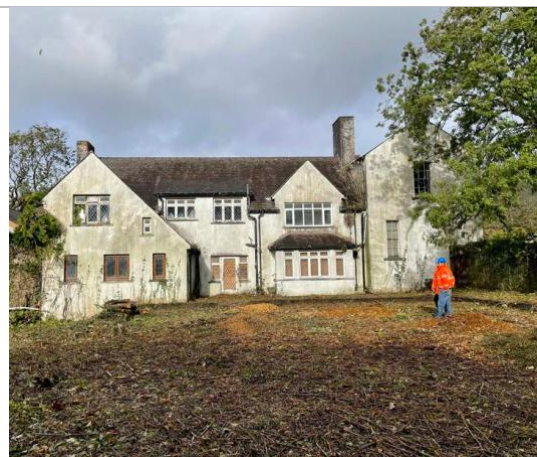
Fig 3. View of the southern facade of Tyn-y-Caeau
