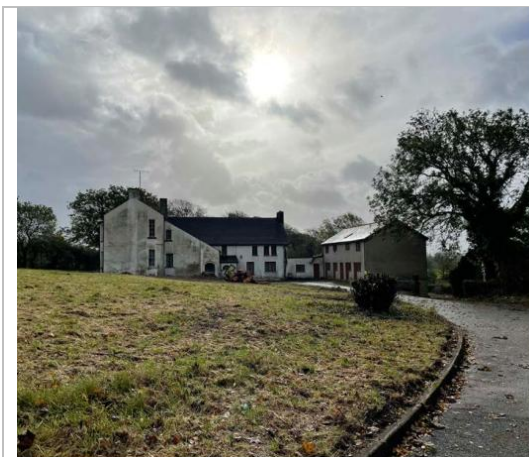
Fig 2. View from the centre of the site, towards Tyn-y-Caeau building, located on the southwest part of the site (PDAS)
