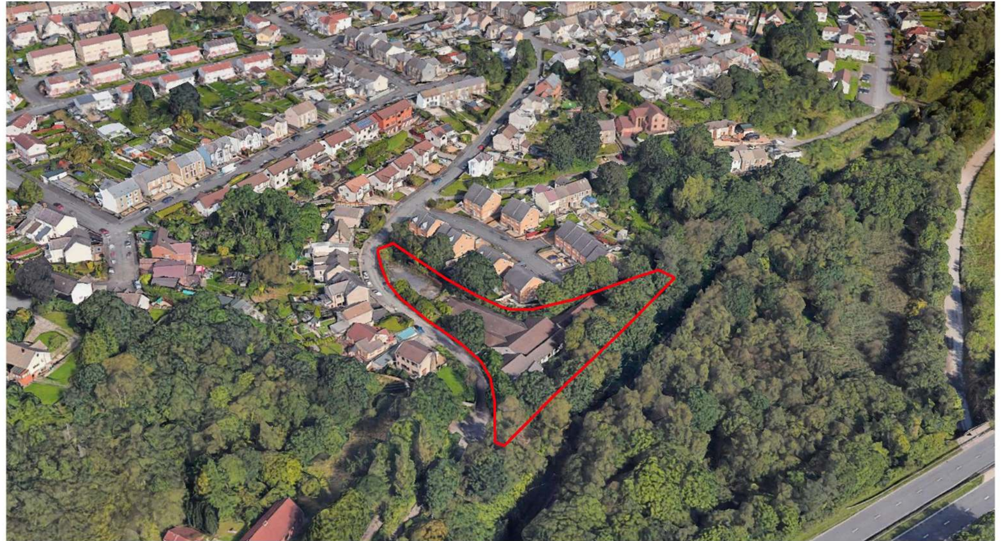
Semi aerial view of the site looking north
