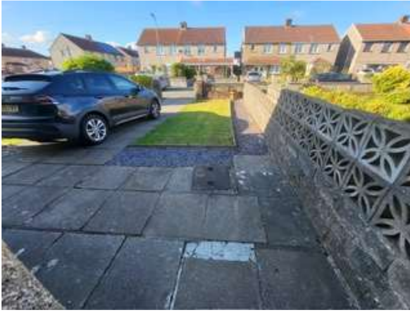
View of other side of front garden area with blockwork walls, lawn and concrete driveway and paths
