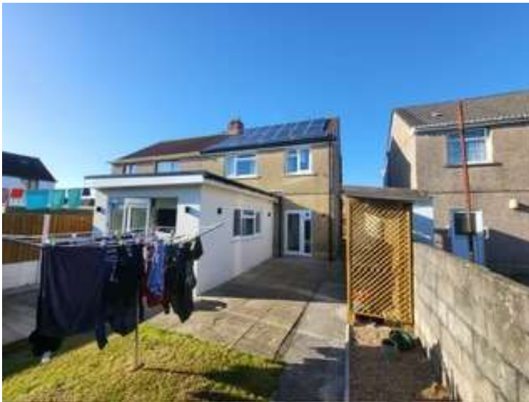
Rear garden area with concrete paving patio areas, blockwork and timber fence panel boundaries. Small lawn to the rear area.
