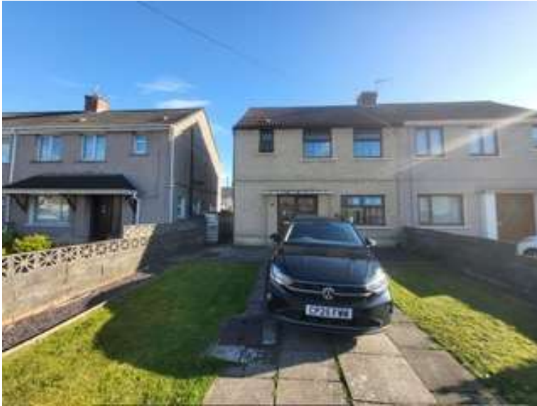
Front garden view showing lawns, concrete driveway and blockwork boundary walls
