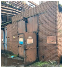
Dust Suppression buildings
