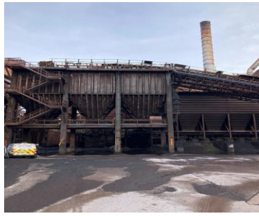
No4 Fines & Coke Bunker
