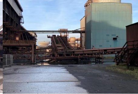
No5 Fines & Coke Bunkers
