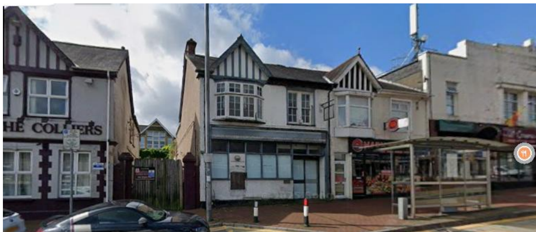
Image 01_ Existing Front View
