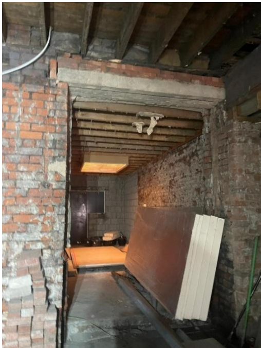
Image 06_ Existing flat roof and rooflight and metal barriers (will be removed)
