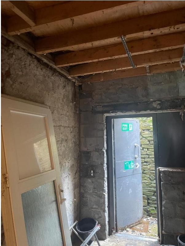
Image 04_ Location of the kitchen and the area designated for the extract duct and ventilation system.
