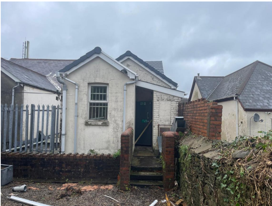
Image 05_ Existing rear view.
