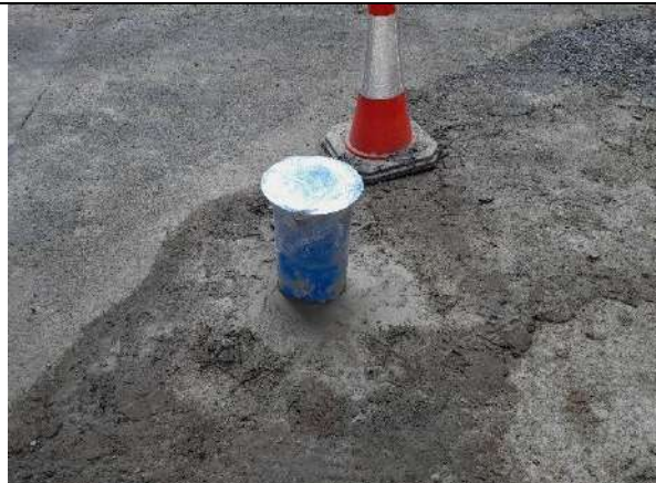
5. Headworks secured on site.
