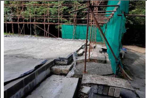
3. General site photograph.
