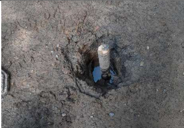
1. Standpipes left proud prior to GGS arrival.
