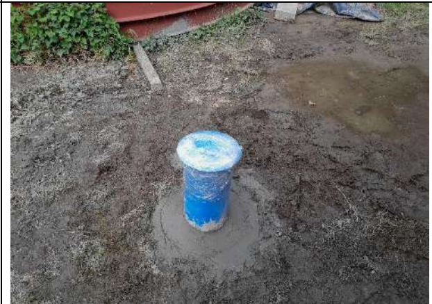
6. Headworks secured on site.
