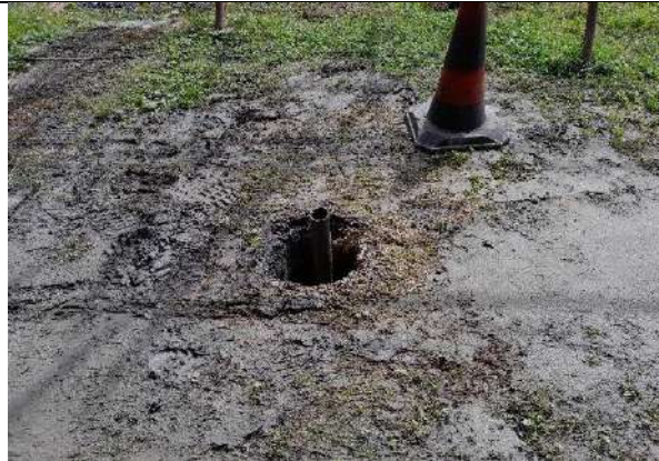
2. Standpipes left proud prior to GGS arrival.
