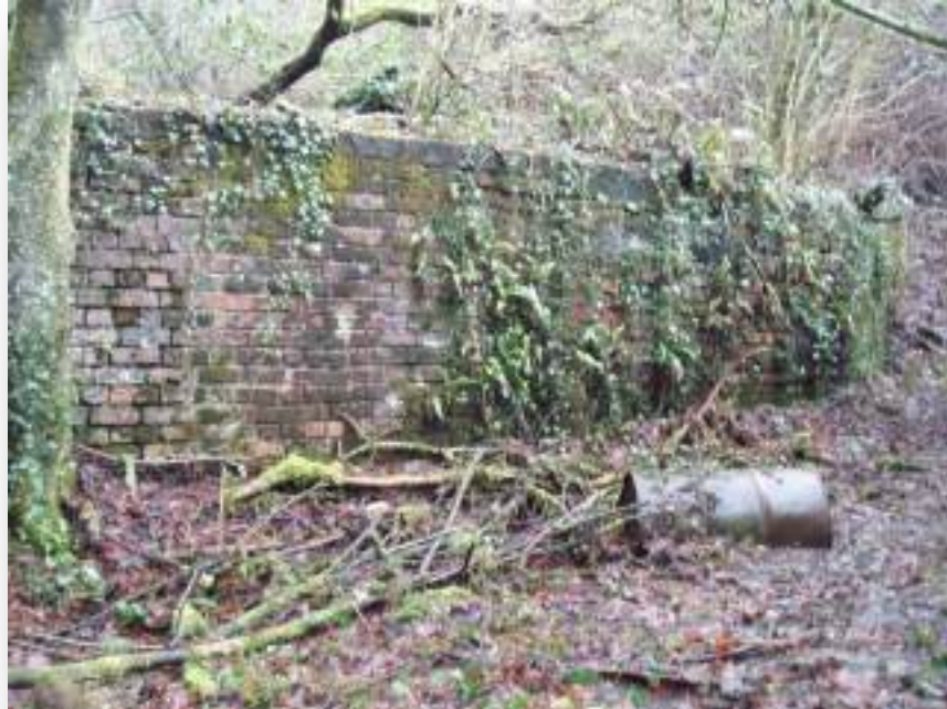
Figure 7 Brick Ventilation Tunnel Adjacent to Adit 277209-058
