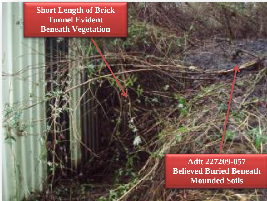
Figure 10 Convergence of Brick Tunnel from Adit 277209-060 with Adit 277209-057
