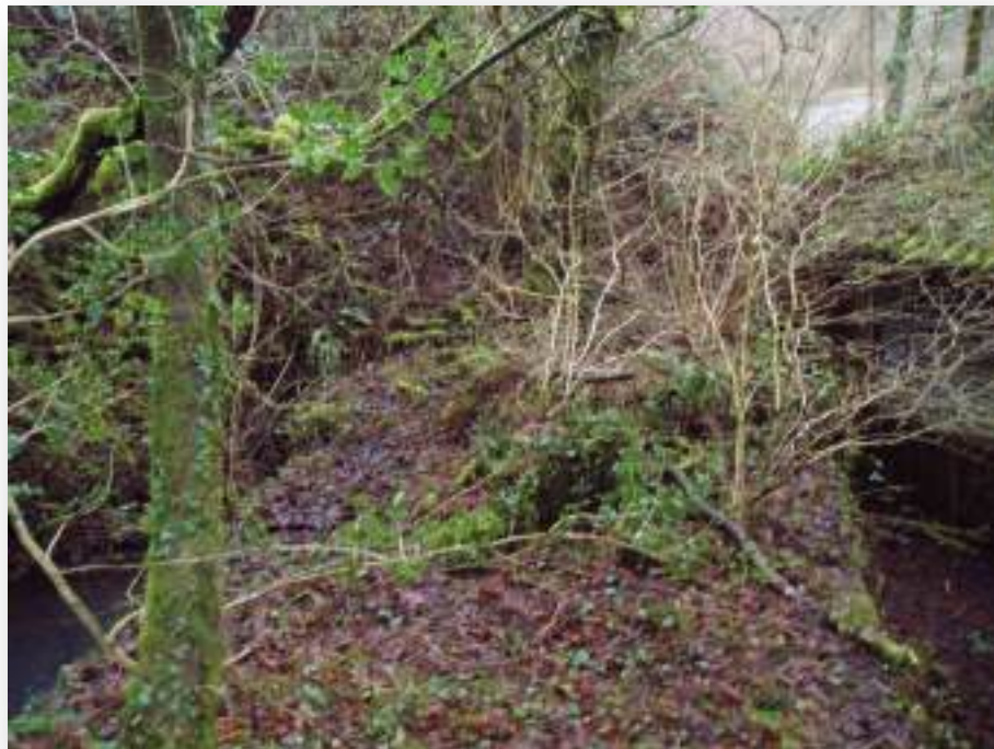
Figure 8 Brick Ventilation Tunnel Adjacent to Adit 277209-058
