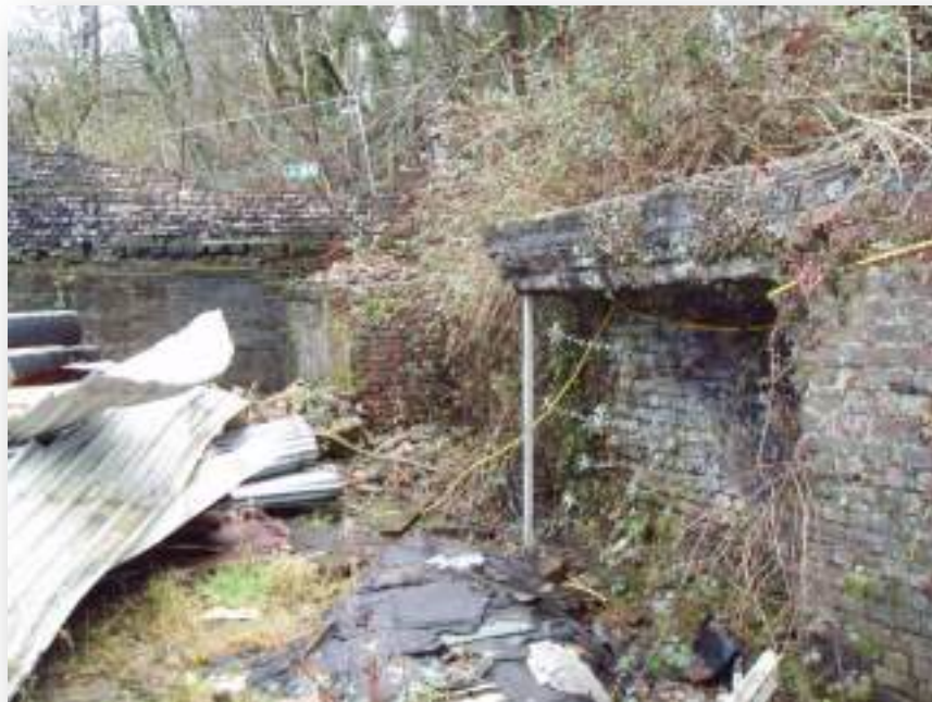
Figure 6 Brick Ventilation Tunnel Adjacent to Adit 277209-057
