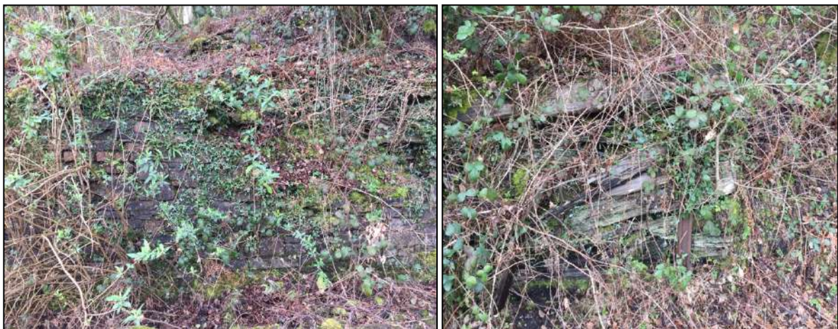
Figure 11. Short sections of stone wall and sleepers used as retaining wall
