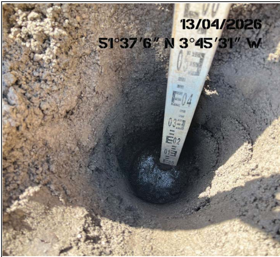
Plot 15 Membrane Placement at Base of Soils
