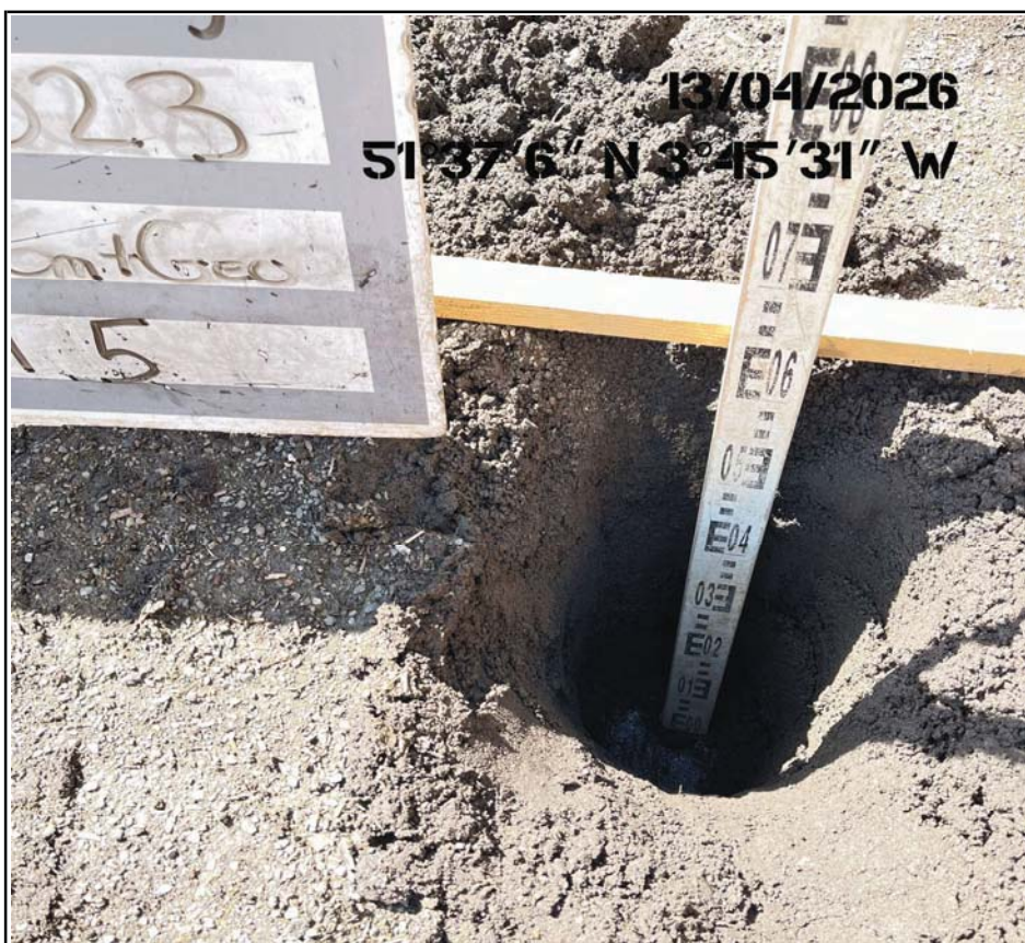
Plot 15 Capping Depth Check Soils
