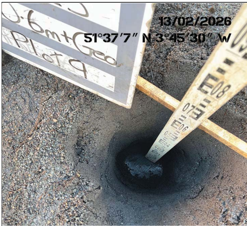
Plot 9 Excavation Showing Membrane Placement
