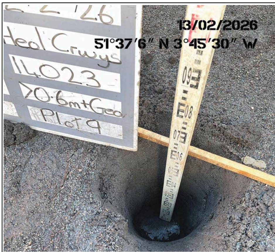
Plot 9 Trial Pit Excavation
