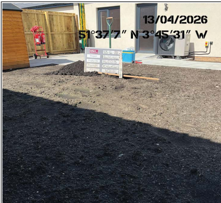
Plot 10 Capping Depth Check Soils
