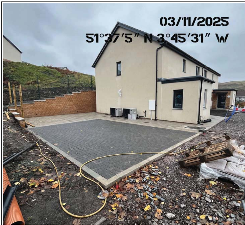
Plot 40 to 43 Parking Bays to The West of the Unit
