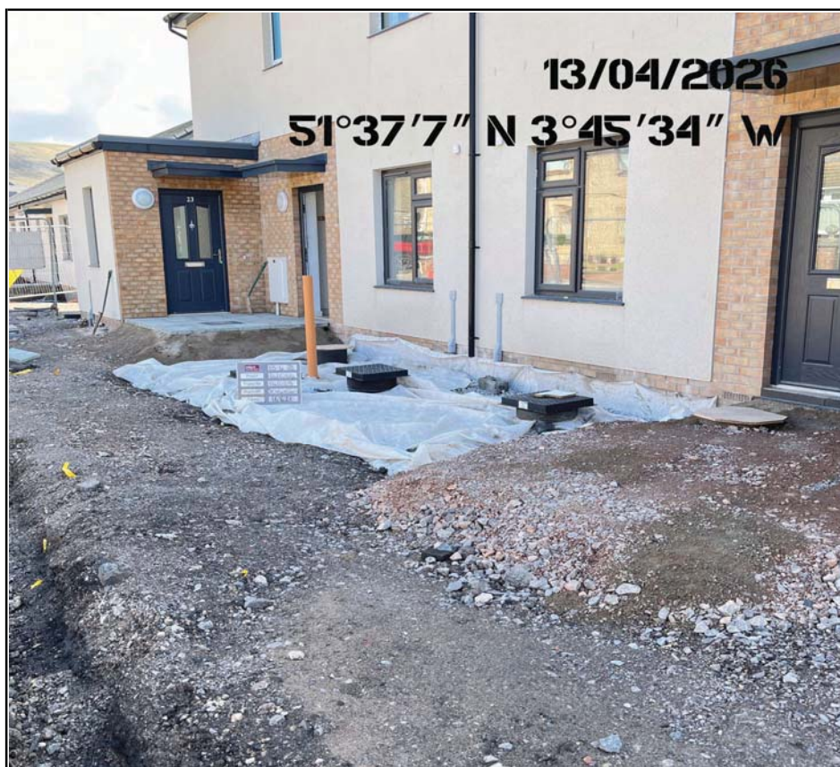
Plot 16 to 21 Rain Garden System (Under Construction)
