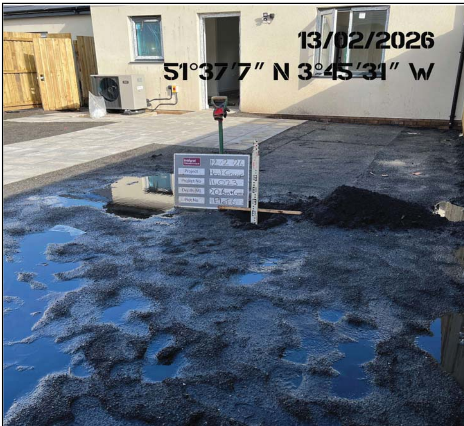
Plot 6 Capping Depth Check
