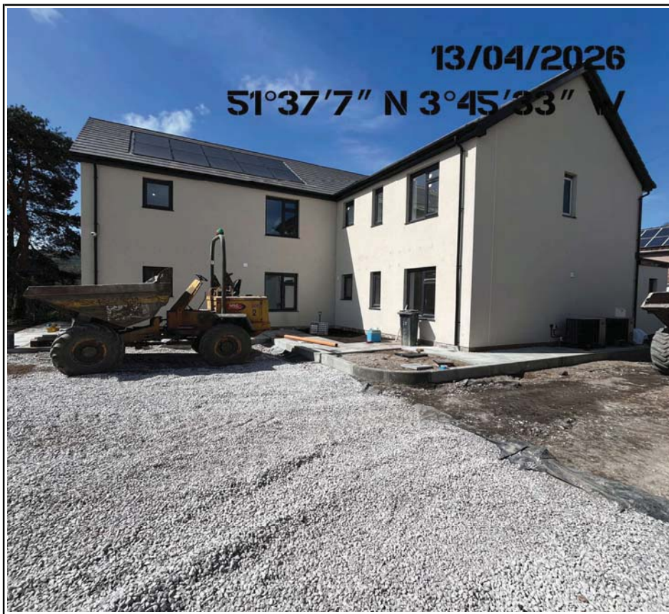
Plots 16 to 21 Car Parking Areas (Under Construction)
