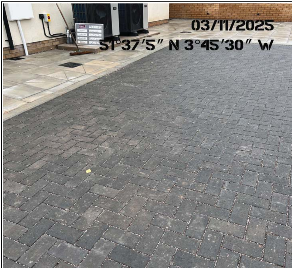
Plot 40 to 43 Permeable Paving Blocks East Area
