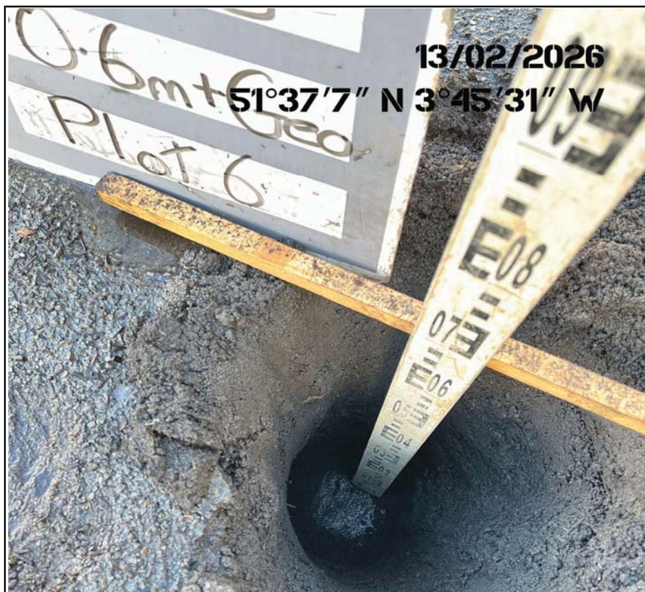
Plot 6 Excavation Showing Membrane Placement
