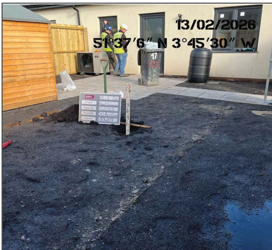
Plot 9 Capping Depth Check
