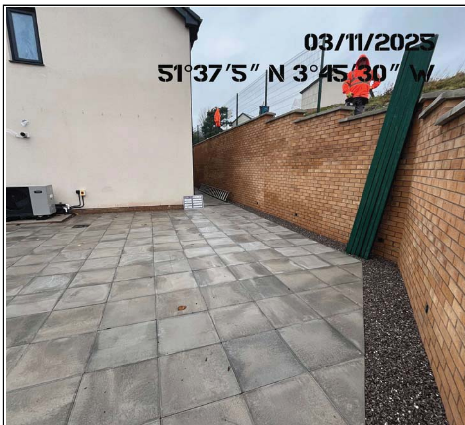
Plot 40 to 43 Hard Finished Patio Slabbed Areas Continuing Around the Rear of the Residential Unit.
