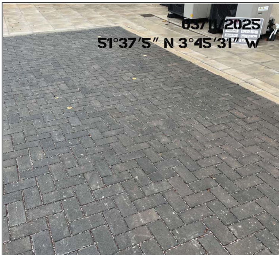
Plot 40 to 43 Permeable Paving Blocks West Area
