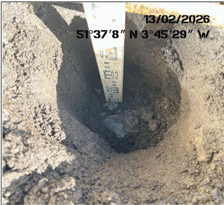
Plot 1 to 4 POS Area Excavation Membrane Placement
