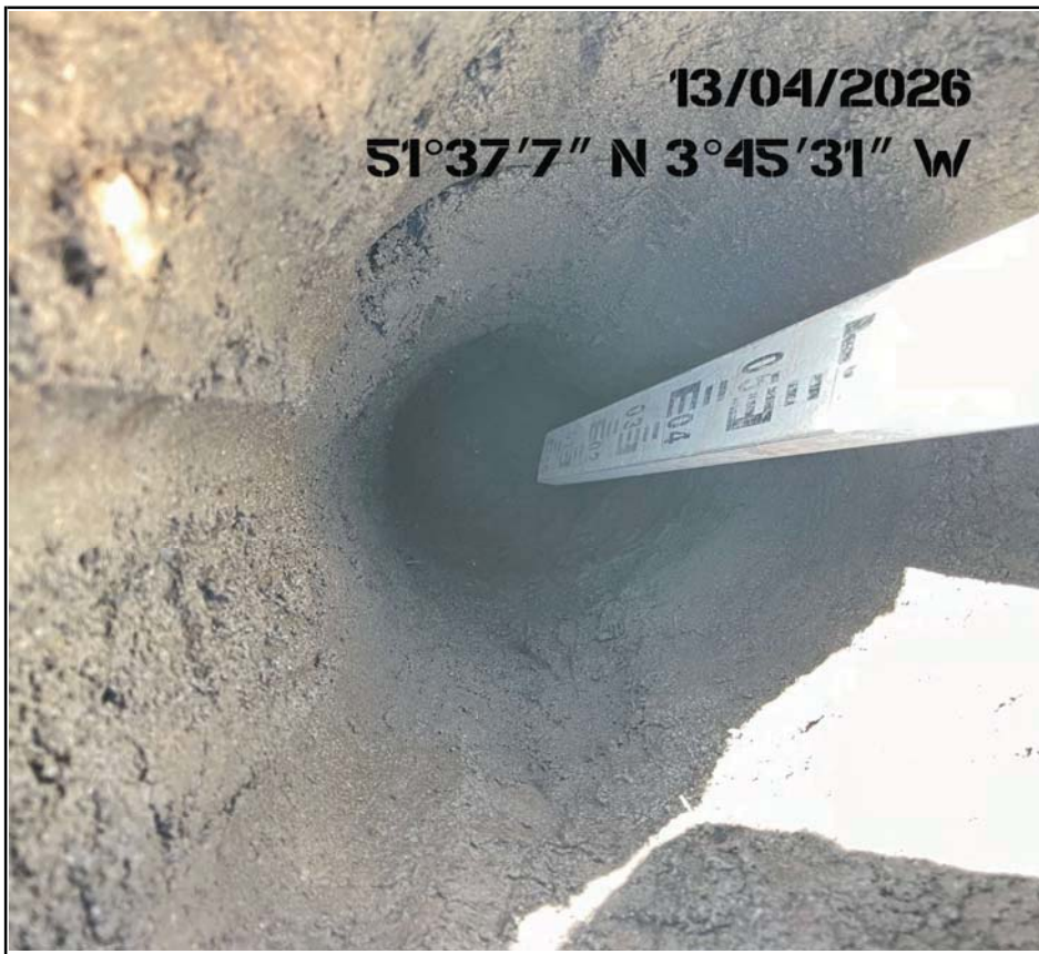
Plot 10 membrane Placement at Base of Soils
